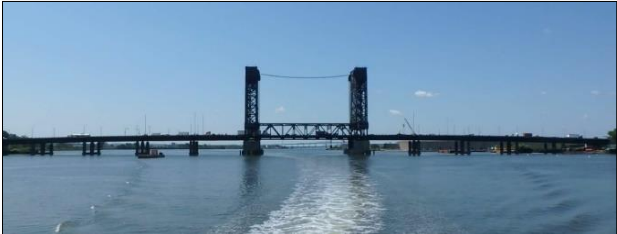
Photo 1: Rt. 1&9T over the Hackensack River as viewed from the river.
