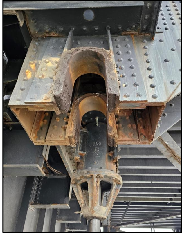
Photo 4: Left - Live Load Shoe Fixed Pin; Right - Live Load Shoe Saddle
