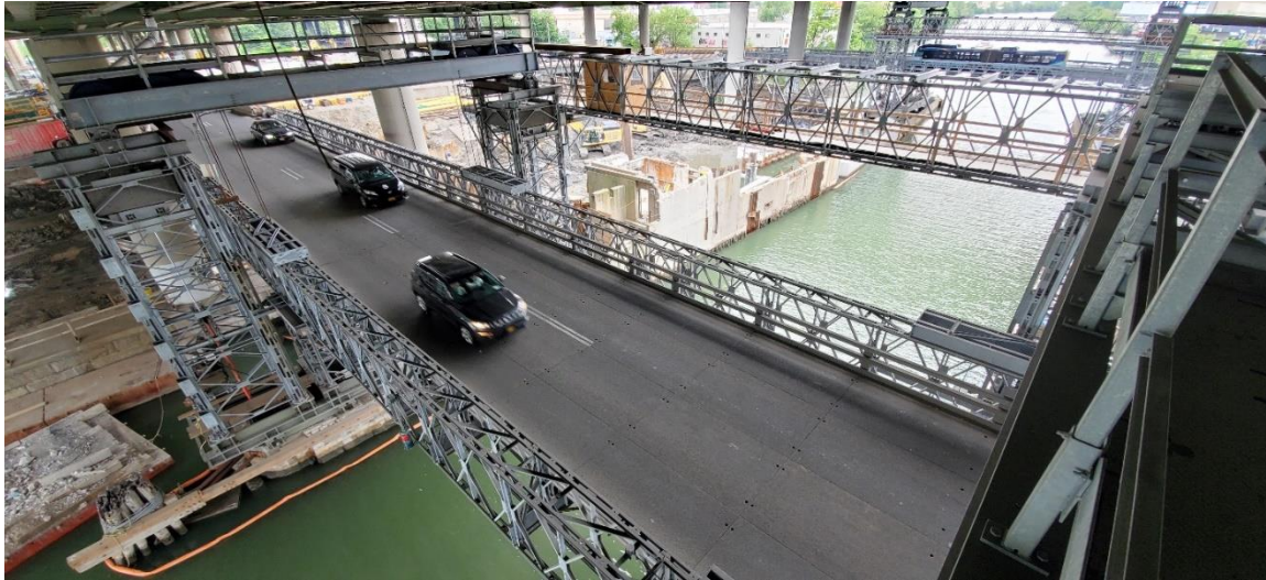
Unionport Temporary Lift Span
