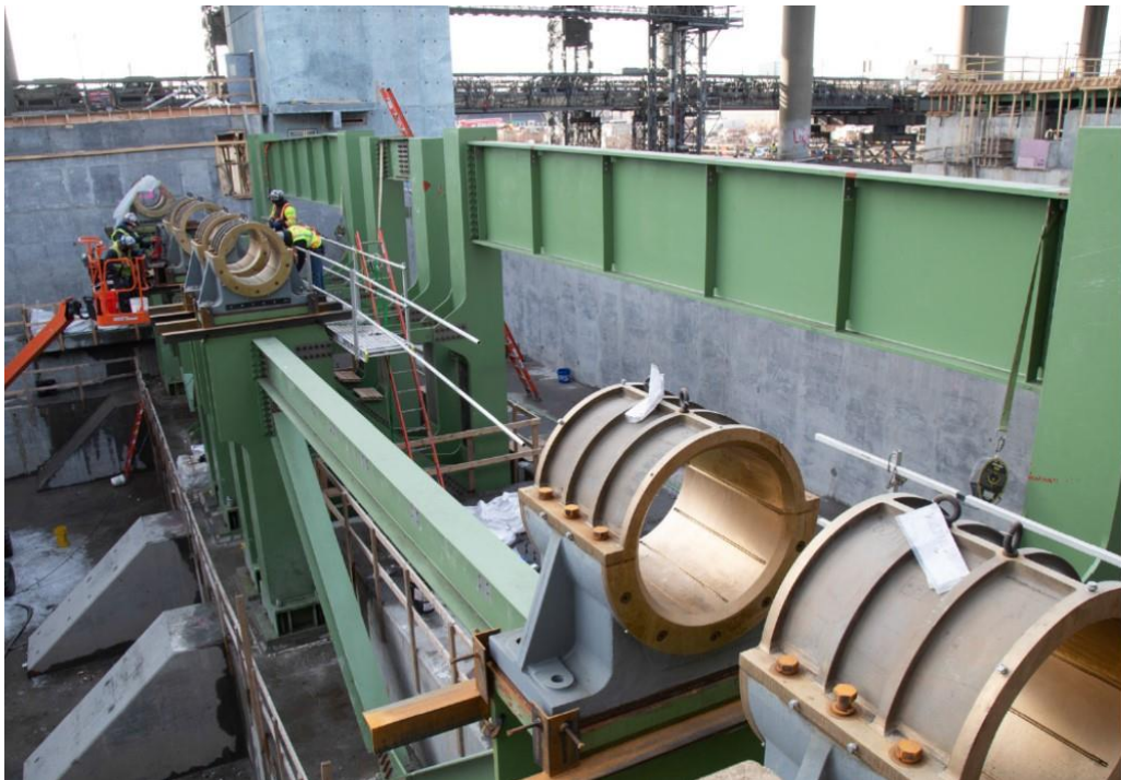
Bascule Span Trunnion Bearing Installation
