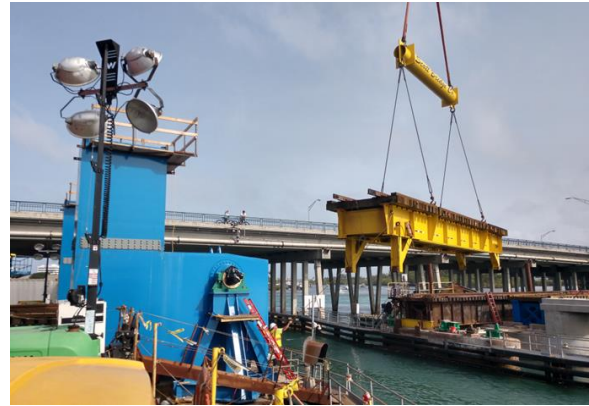
Flying jump span being removed from the channel
