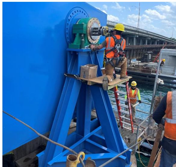
Checking trunnion alignment after setting counterweight girders on towers
