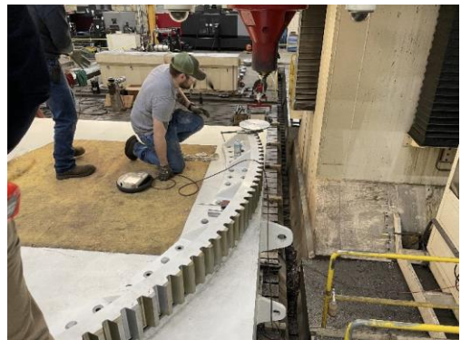
Checking rack alignment on the mill
