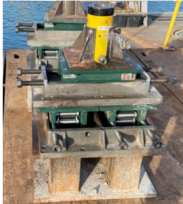
Manipulator to aid alignment of toe section
