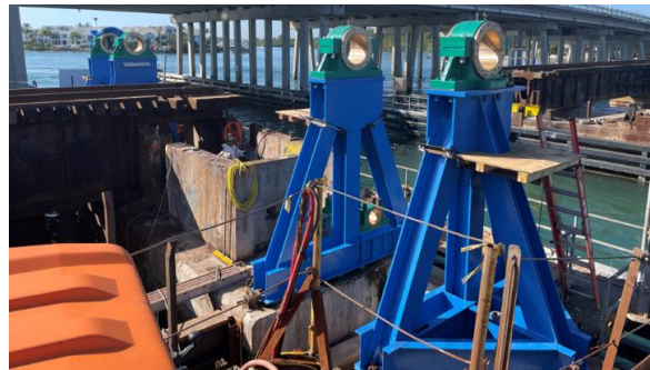
Towers installed and aligned on pier
