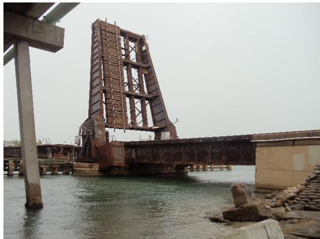
Existing Bascule Span in the Raised Position
