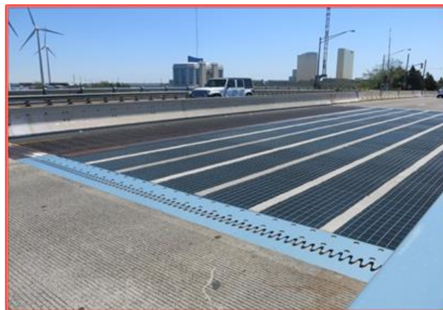
Figure 7: Stage 1 Finished Steel Open Grid Deck
