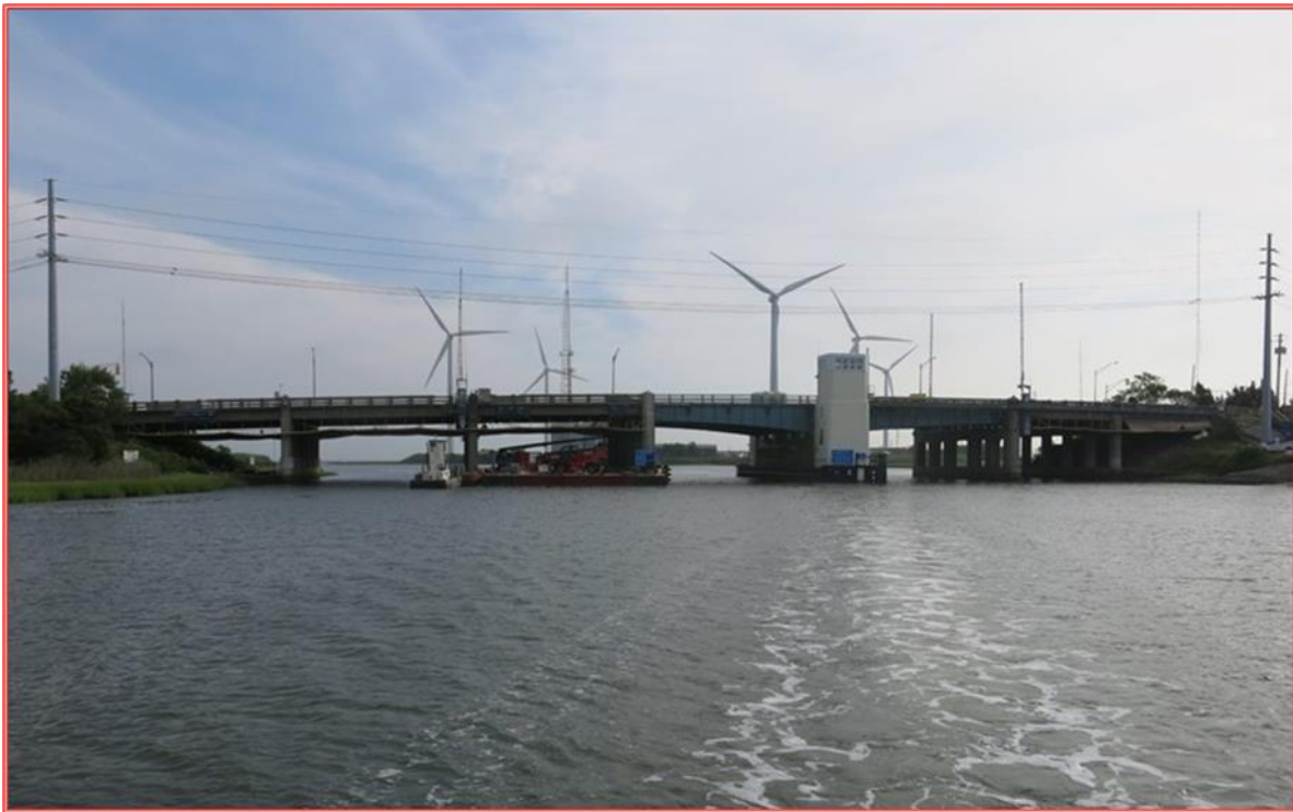
Figure 1: Rt. 30 over Beach Thorofare Bridge
