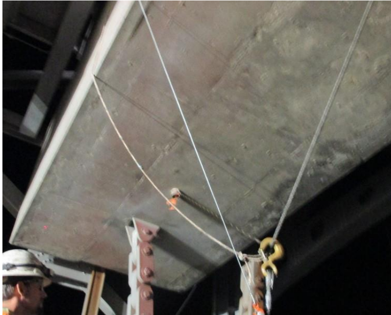
Figure 3: Counterweight pulled down with a winch to raise the movable span.
