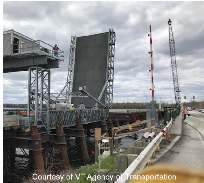
PHOTO 4: Temporary Bridge In The Open Position
