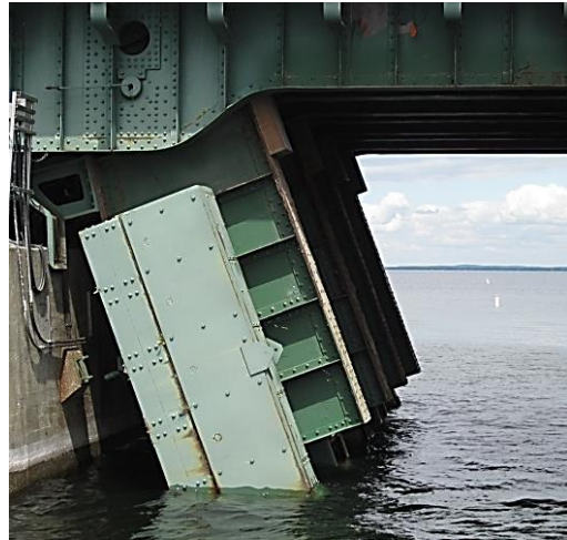
PHOTO 3: Former Span In The Open Position - Note Counterweight Was Partially Submerged In The Water.
