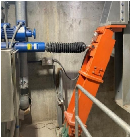
PHOTO 11: Tail Lock Machinery
