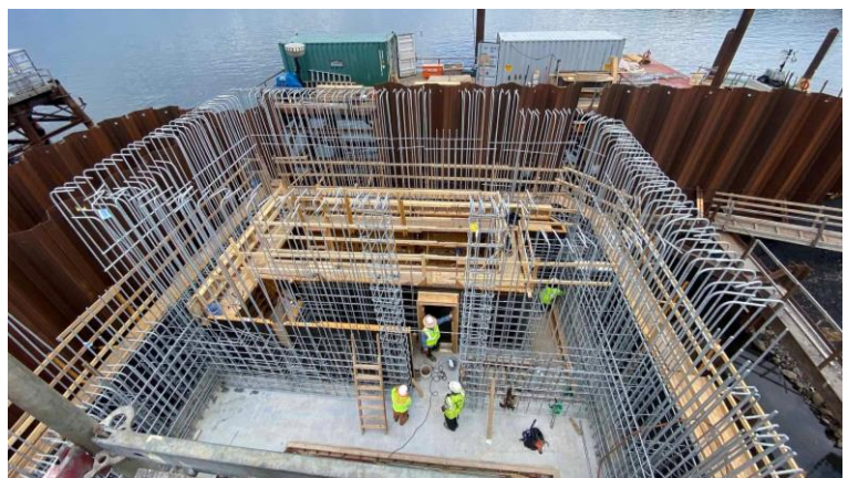
PHOTO 18: Bascule Pier Wall Reinforcement Placement
