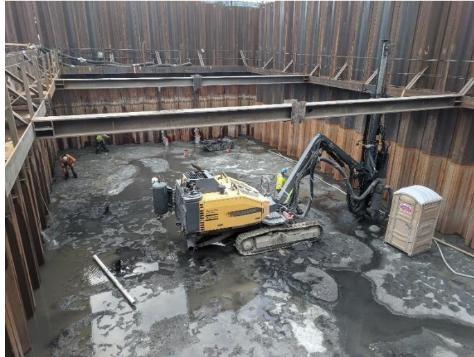
PHOTO 17: Installation of Rock Anchors Through Tremie at Pier 2
