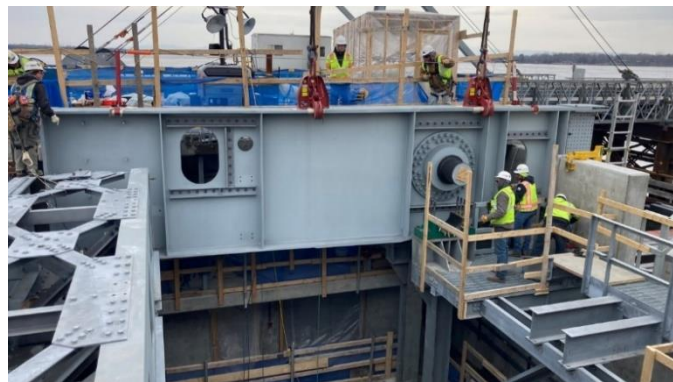
PHOTO 8: Bascule Girder Field Assembly
