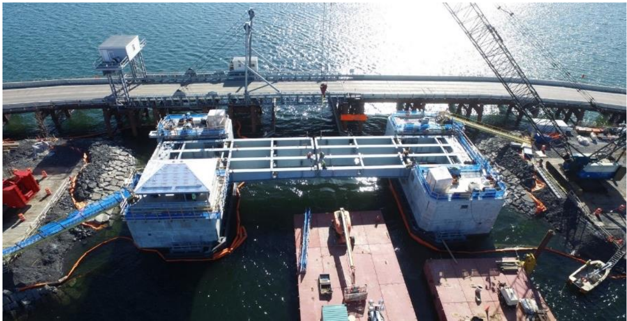
PHOTO 19: Bascule Piers and Leaves Erection
