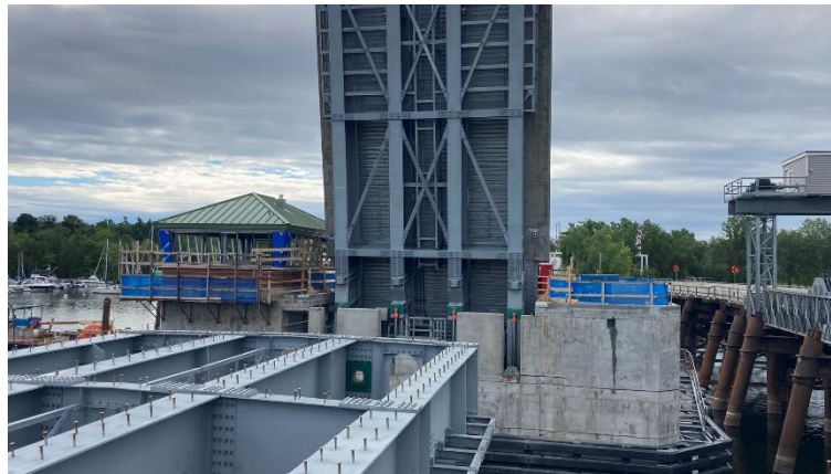
PHOTO 5: Bascule Leaf Framing View
