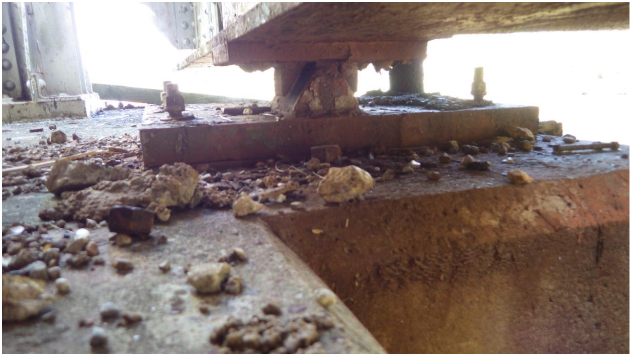
Photo 4 – Lift Span Liveload Bearing
