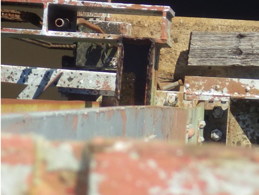
Photo 9 – Northern Tower Legs Appeared to be Bowed Above Base
