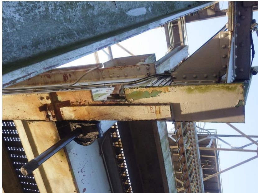
Photo 6 – End Floorbeams Were Torch Cut & 1" Thick Repair Plate Was Welded to NW & SW Sides for Span Locks
