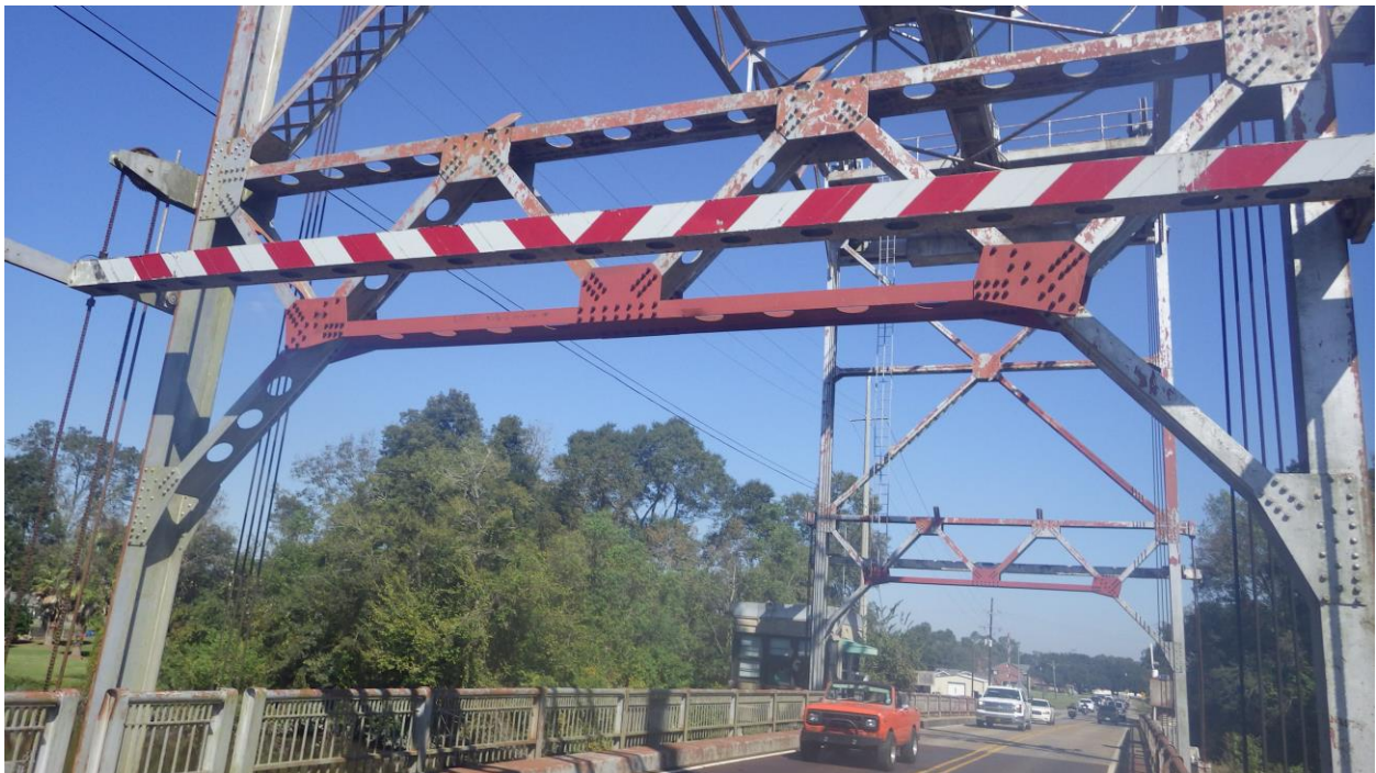
Photo 2 – Tower Portal (replaced due to collision)
