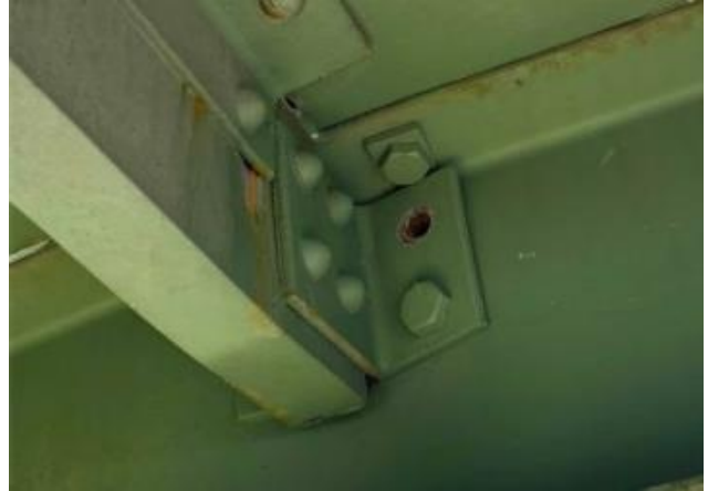
Figure 8: Damage to stringer in line with impact
