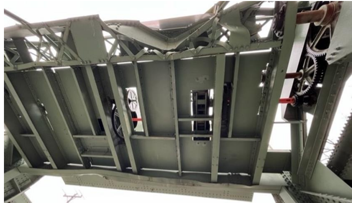
Figure 4: Damage to the machinery platform from below
