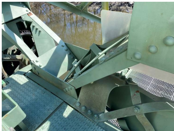
Figure 5: Damage to diagonals
