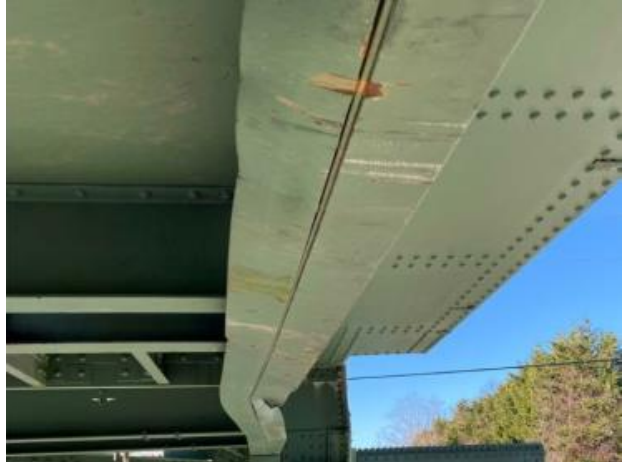
Figure 11: Counterweight girder bottom flange
