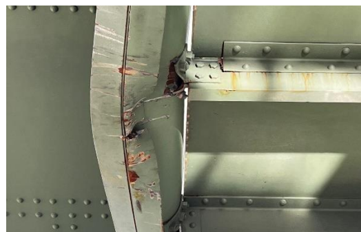
Figure 15: Damage to counterweight girder
