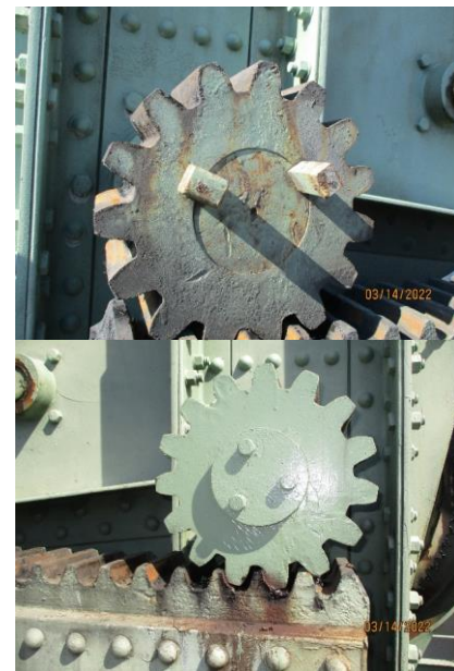
Figure 16: Missing gib head, east (top); cut off keys with cap, west (bottom)
