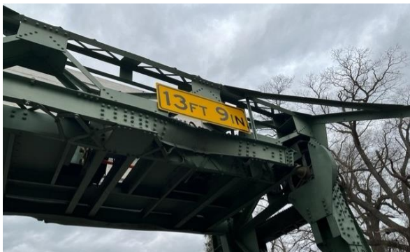
Figure 2: Damage to portal frame from impact
