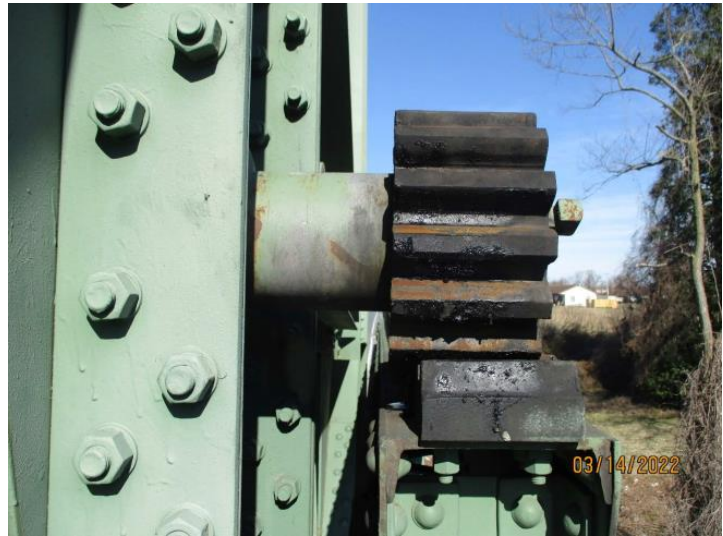
Figure 10: Pinion pulled towards middle of bridge
