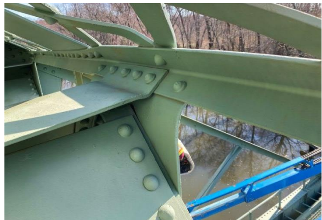
Figure 6: Deformation of upper chord and gussets
