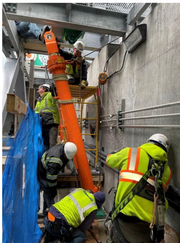
Photo No. 9: Installation of hydraulic cylinders installed on the North Pier.
