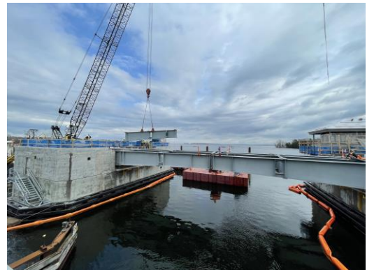
Photo No 7: Erection of the North Bascule steel.
