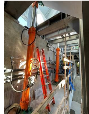
Photo No. 12: North Pier hydraulic cylinders fully extended.
