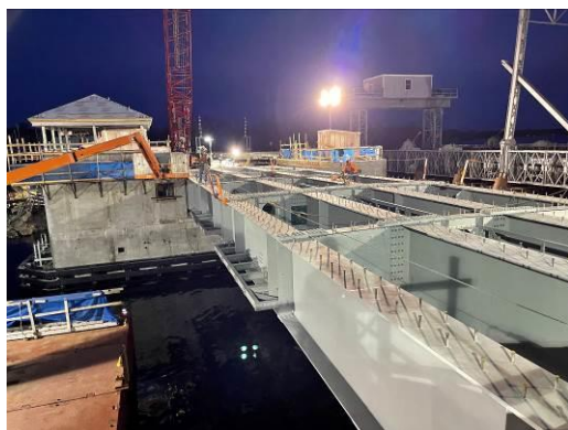
Photo No. 8: North and South Piers bolts being snug tighten during a night shift.
