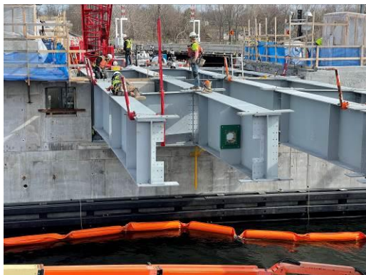
Photo No 6: Erection of the South Bascule steel.
