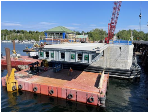
Photo No. 13: Completed steel and deck on the South Bascule Span with leaf in the lowered position.
