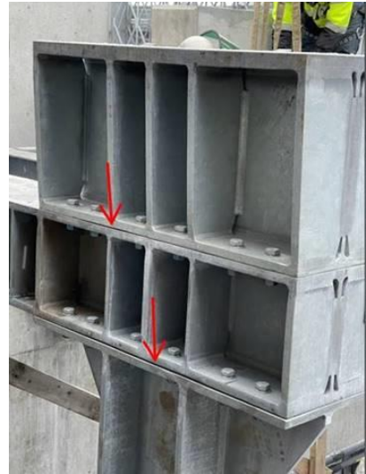
Photo No. 4: Steel gaps in the trunnion support are shown.
