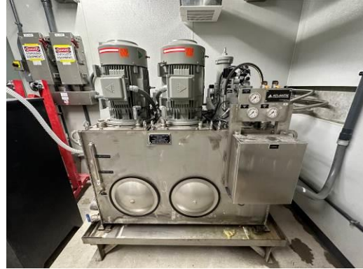
Photo No. 16: North Hydraulic power unit in the pier's machinery room.
