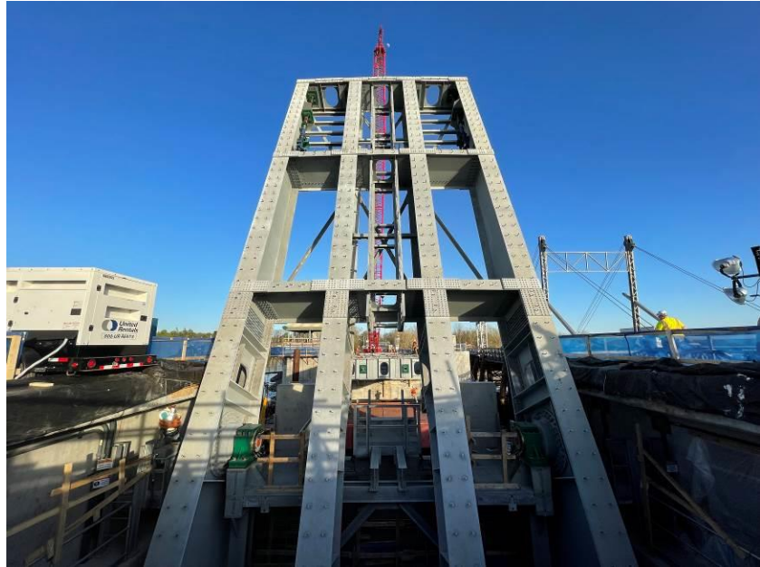
Photo No. 10: North Pier partially assembled in the open position.
