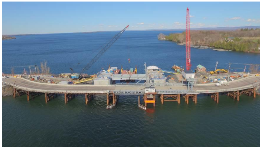
Photo No. 2: The North Hero Movable Bridge Construction site with the temporary bridge adjacent to the new hydraulic bascule bridge.
