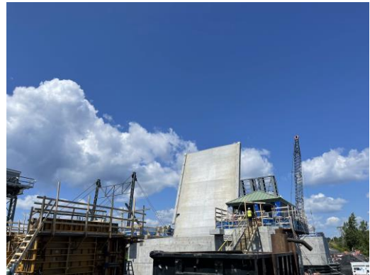
Photo No. 14: Completed South Bascule Span in the upright position with the incomplete North Bascule Span open in the background.
