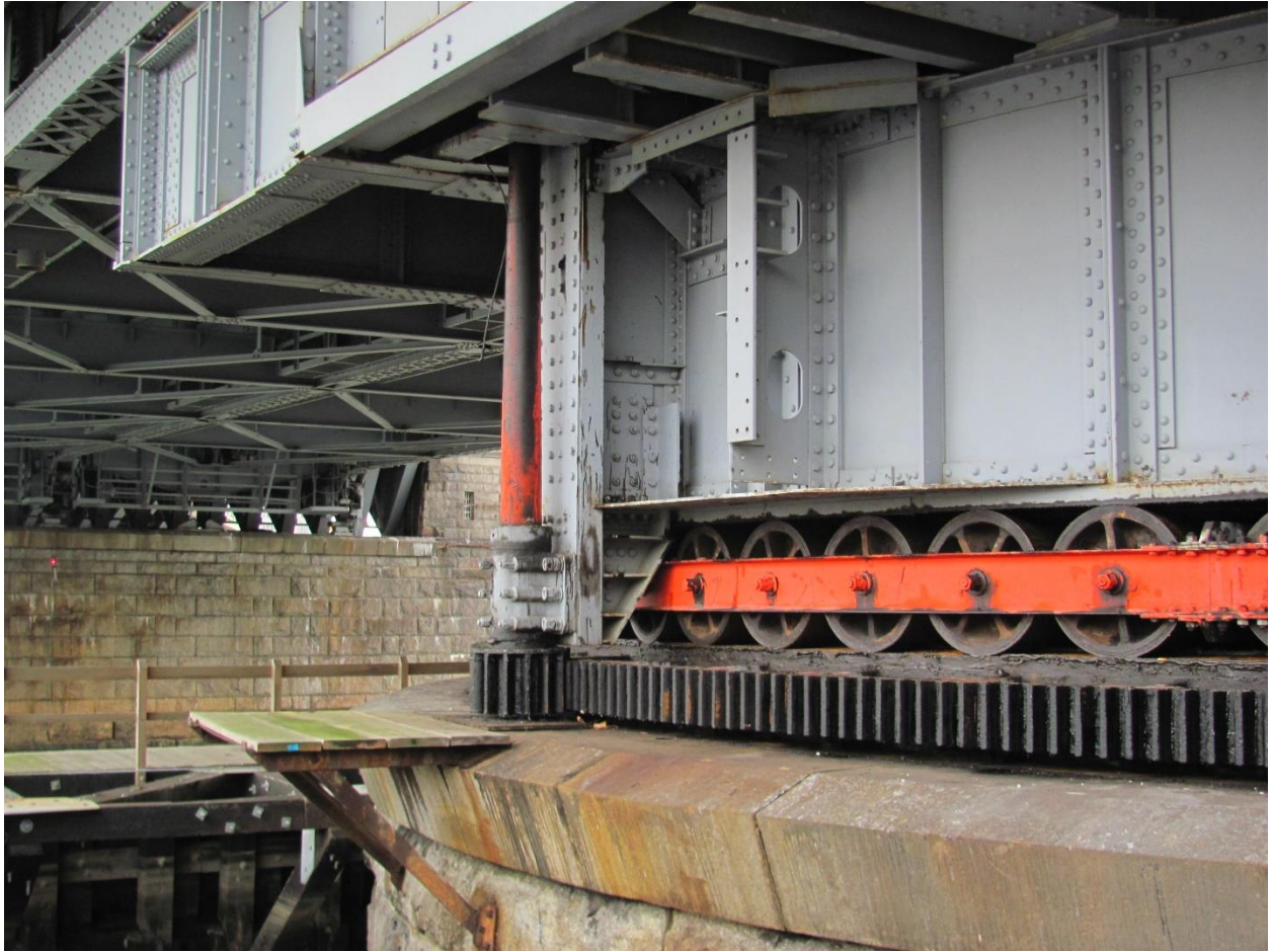
CAPTION: Existing rack, north pinion and center pier with small platform at the pinion location and no railing.
