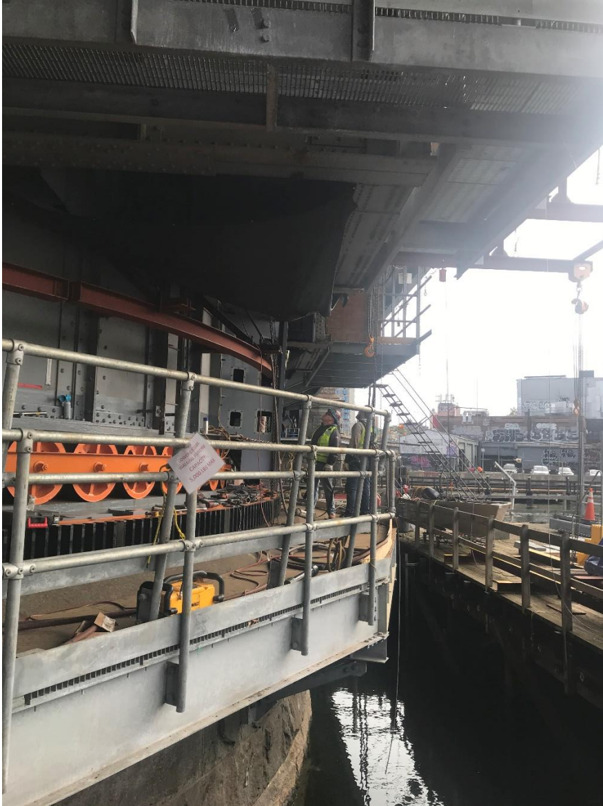
CAPTION: New access platform around the center pier for maintenance and inspection of the rack, pinions, rollers and tracks.
