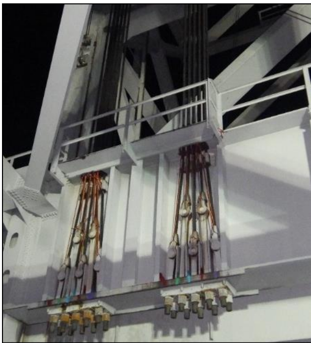
Figure 6: Photo of the main counterweight take-ups connecting the wire ropes at the lifting girder. Note the color coding.
