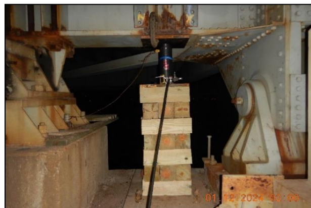
Figure 22: 50-ton jacks under the floorbeam of the opposite end of the rope replacement.
