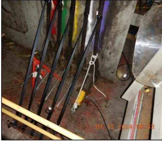
Figure 23: Hydraulic jack and jacking chair used for removing pins at the counterweight.
