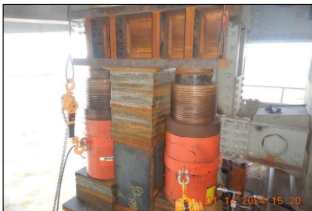
Figure 21: 400-ton jacks under the floorbeam on the rope replacement end of the lift span.
