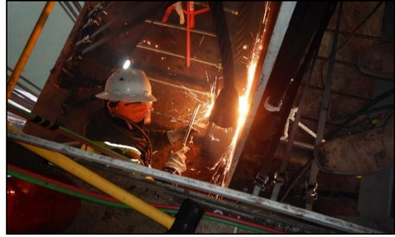
Figure 30: Flame cutting the first main counterweight pin.
