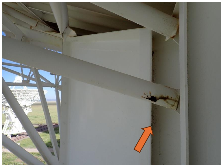
Photo 9 Damage to the Reflector Backup Structure
