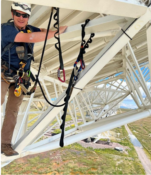
Photo 6 An Inspector using TARA Methods
