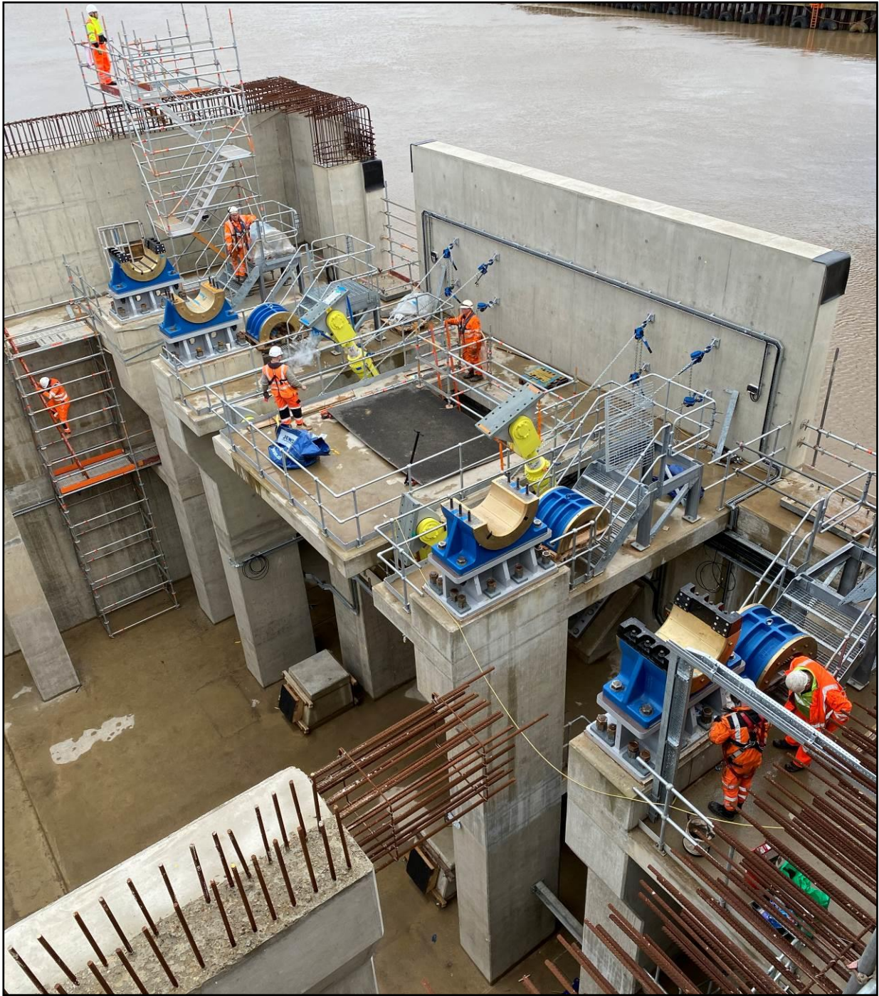
Figure 7 – West Bascule Pier Prior to Crane Placement of the Bascule Span
