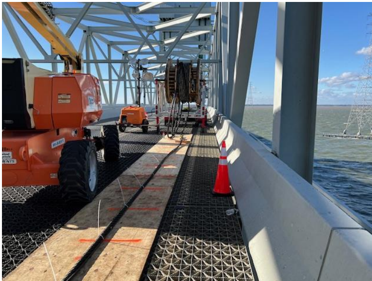
Figure 11: Counterweight ropes pulled off the shipping reel in preparation for installation with a winch.
