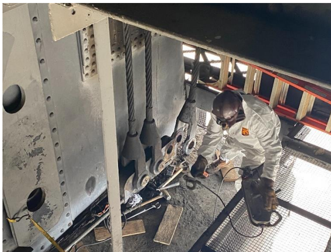
Figure 6: The counterweight end pins are seized and nuts are welded on to remove the pins with jacks.
