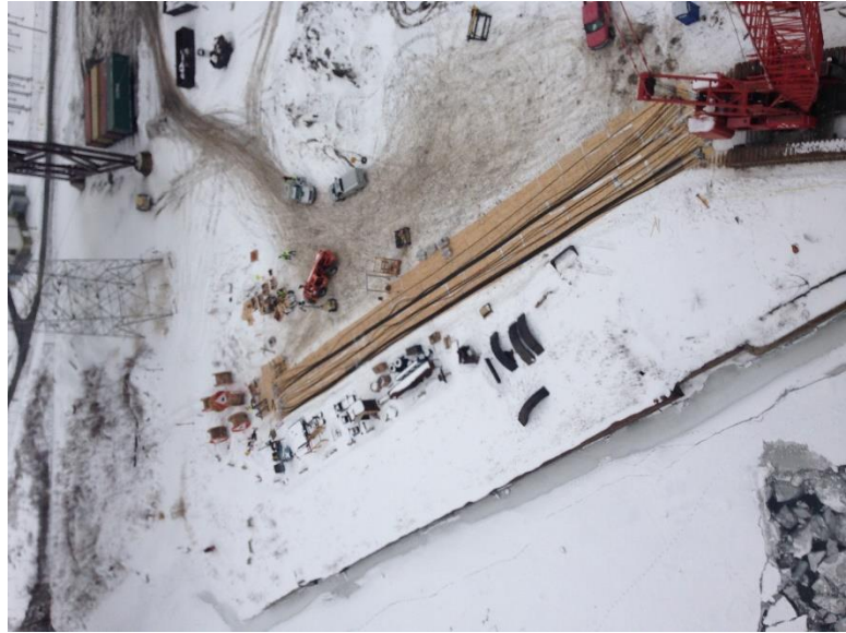
Figure 12: Counterweight ropes pulled off the shipping reel in preparation for installation with a crane.
