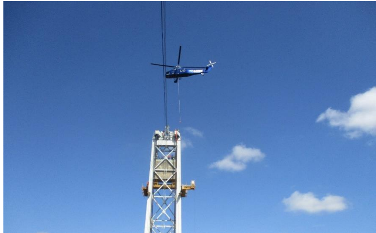
Figure 10: Counterweight rope installation with a helicopter.
