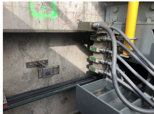
Photograph 8 – Limit switches
