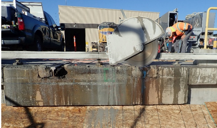
Photograph 15 – A small amount of the west pit wall is being trimmed off
