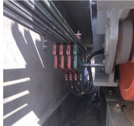
Photograph 5 – New conductor bar system
