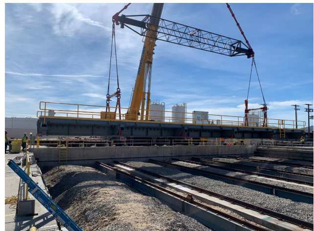
Photograph 14 – Fully assembled transfer table being set into position in the pit at West Colton
