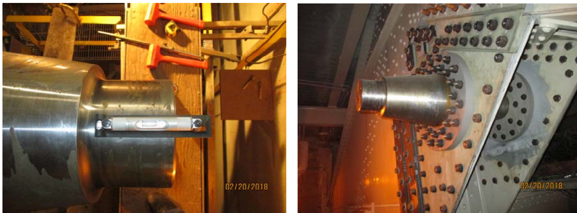
Figure 8 – Alignment Verification and Final Bolting of TOS assembly.
