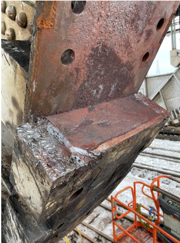
CAPTION: Top photo show excavation of the added weld at the tread joints. Second photo shows joint after one tread section is removed, showing the depth of the added weld.
