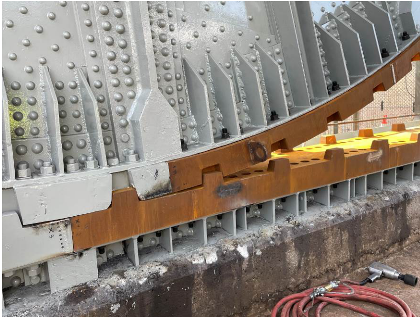
CAPTION: New rear tread and track (unpainted) installed during adjacent to the old tread and track segments (painted grey). Note the modifications to the new tread pockets and the modifications required to old pockets for temporary operation.
