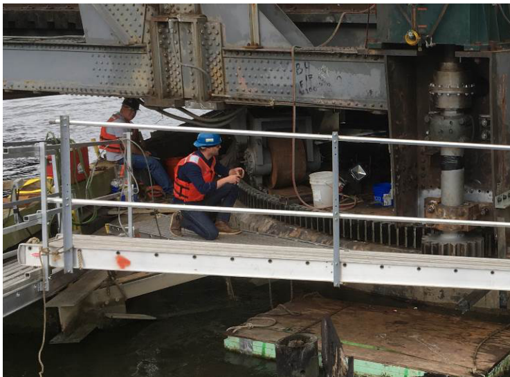
CAPTION: Bogie design allows for access between the four bogies by eliminating the continuous drum girder.
