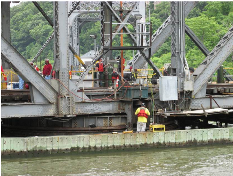
CAPTION: Spuyten Duyvil with old drum girder in place blocking access to pivot pier.
