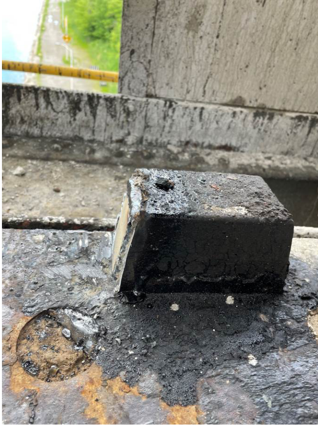
CAPTION: Temporary alignment fix included the addition of ¼ inch plate welded to the old lug to properly align the span at the toe end.
