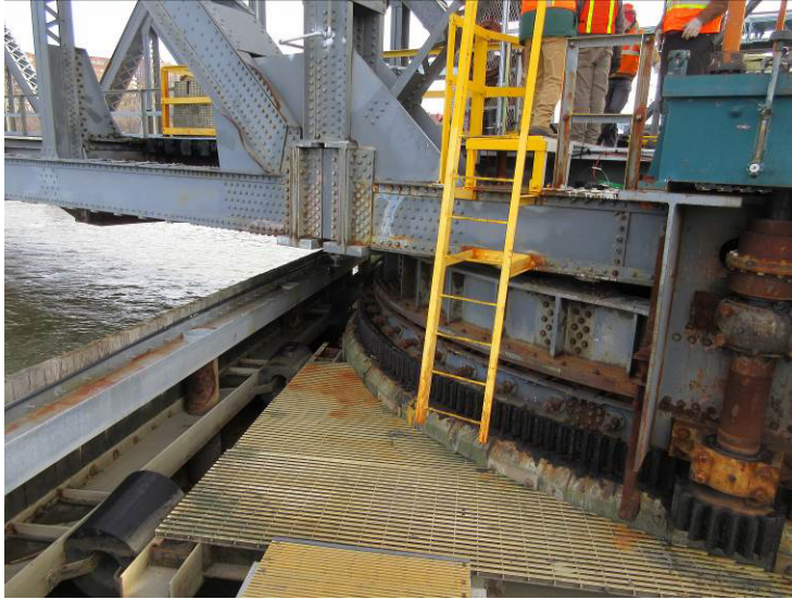
CAPTION: Original drum girder in position blocking off all access to the center pivot pier for routine maintenance.
