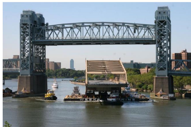
General elevation looking south showing lift span in raised position to allow passage of a marine vessel
