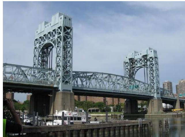
General elevation of Harlem River Lift Span looking southwest
