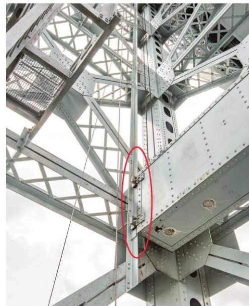
Innovative solutions were developed prior to bid such as proposing lubrication free guides for the counterweights.
