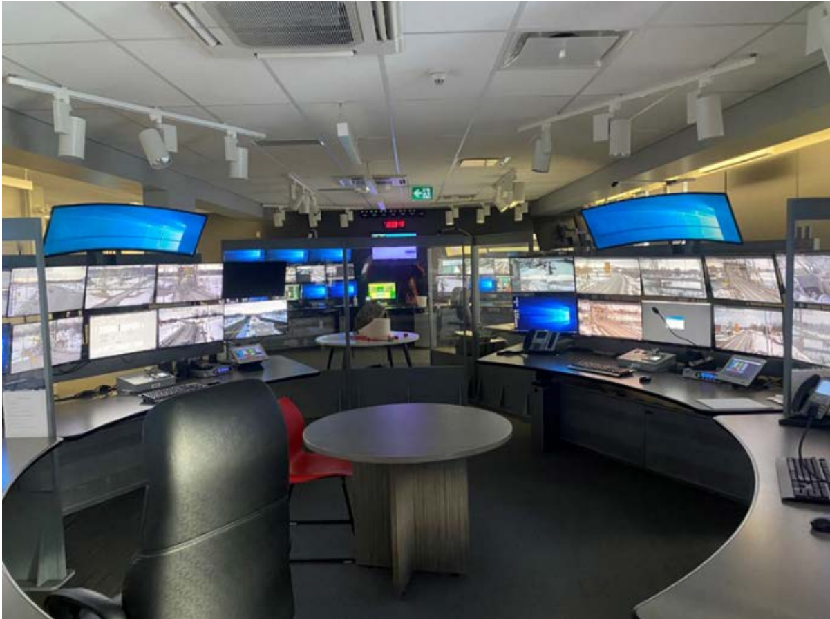
Figure 3 - Operations Control Center
