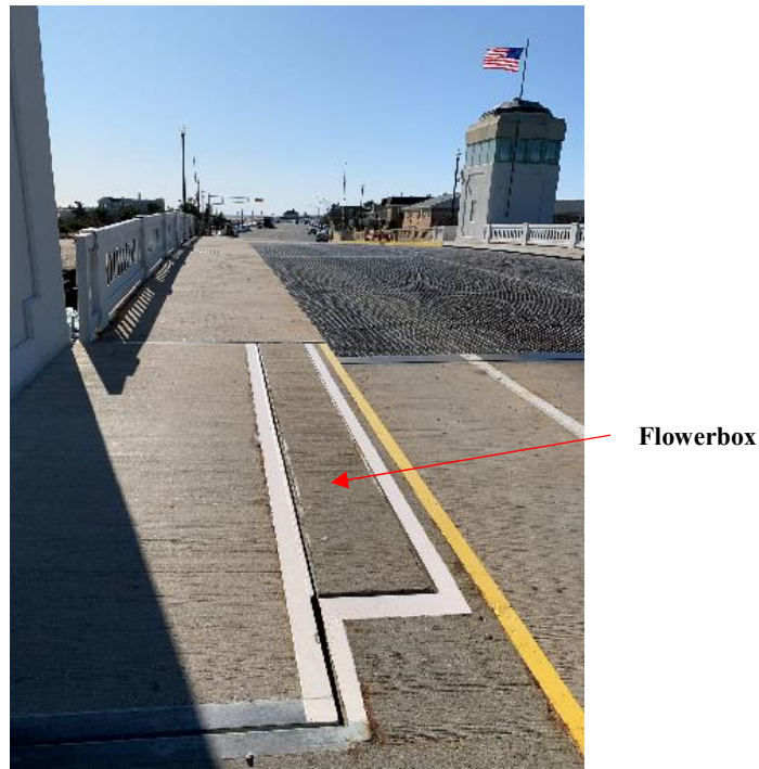
Figure 7 - Flowerbox Opening (Northeast Corner)
