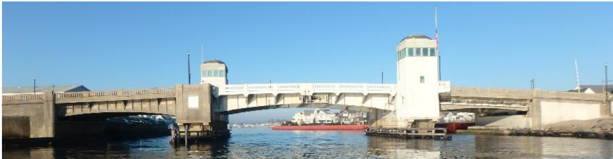
Figure 1 - Bridge W-43 (Looking West)
