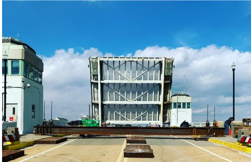
Figure 12 - Strongback Girder following Installation on Southern Span
