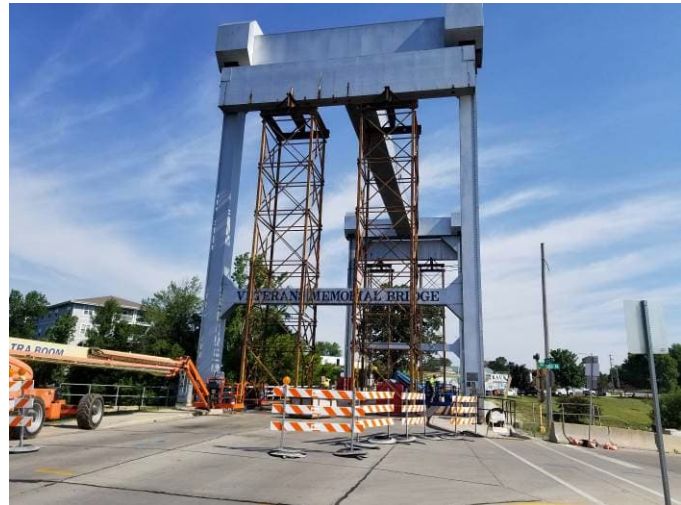
Counterweight shoring for wire rope replacement
