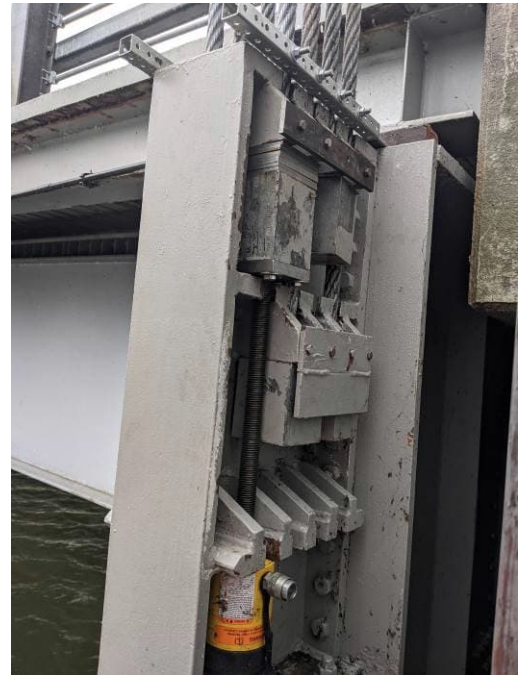
Jacking and shimming new wire rope
