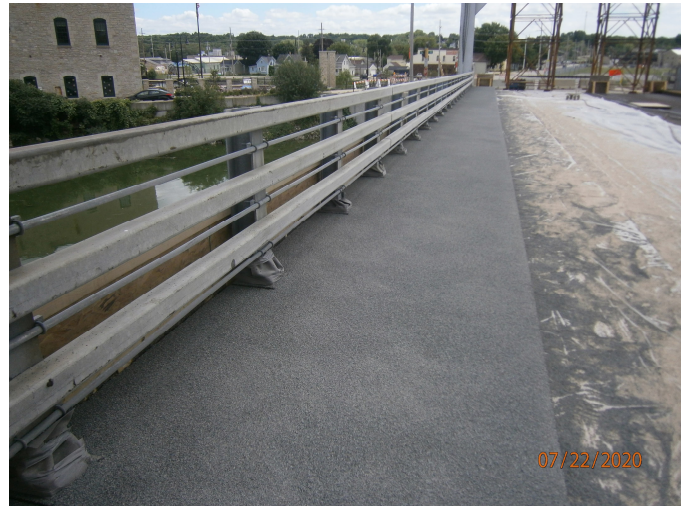
Railing modifications and sidewalk overlay
