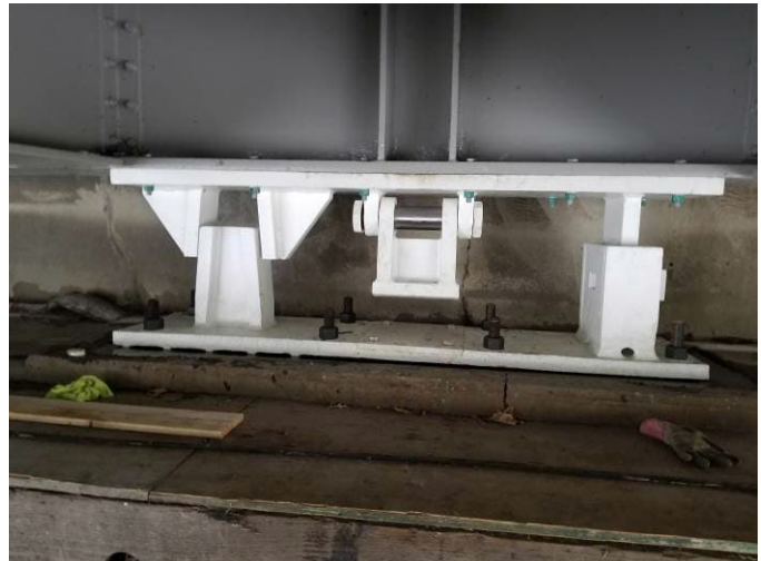
Refurbished alignment guide, rocker bearing & span lock receiver
