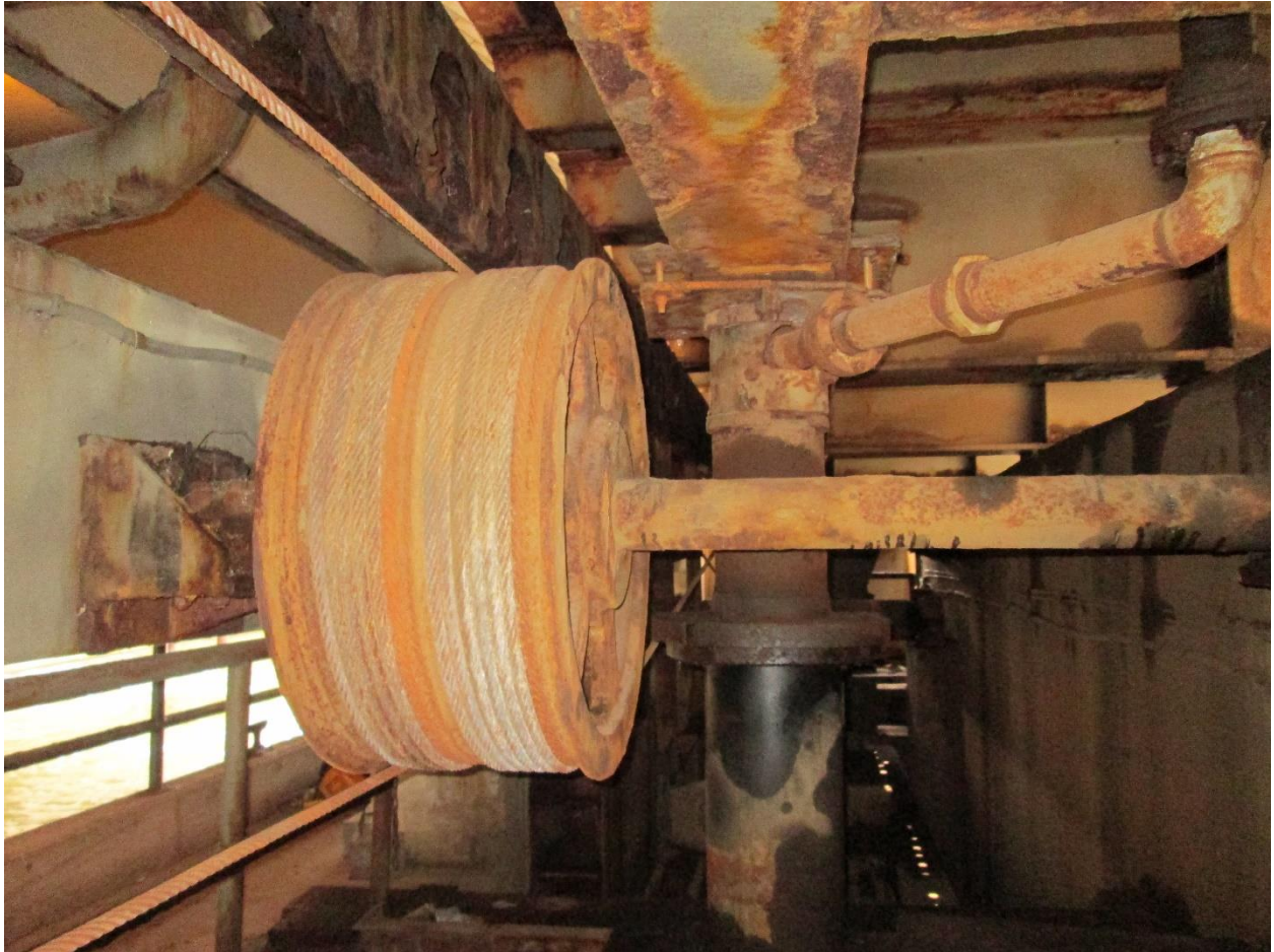
Photo 5: Existing Equalizer Drum and Hydraulic Cylinder.
