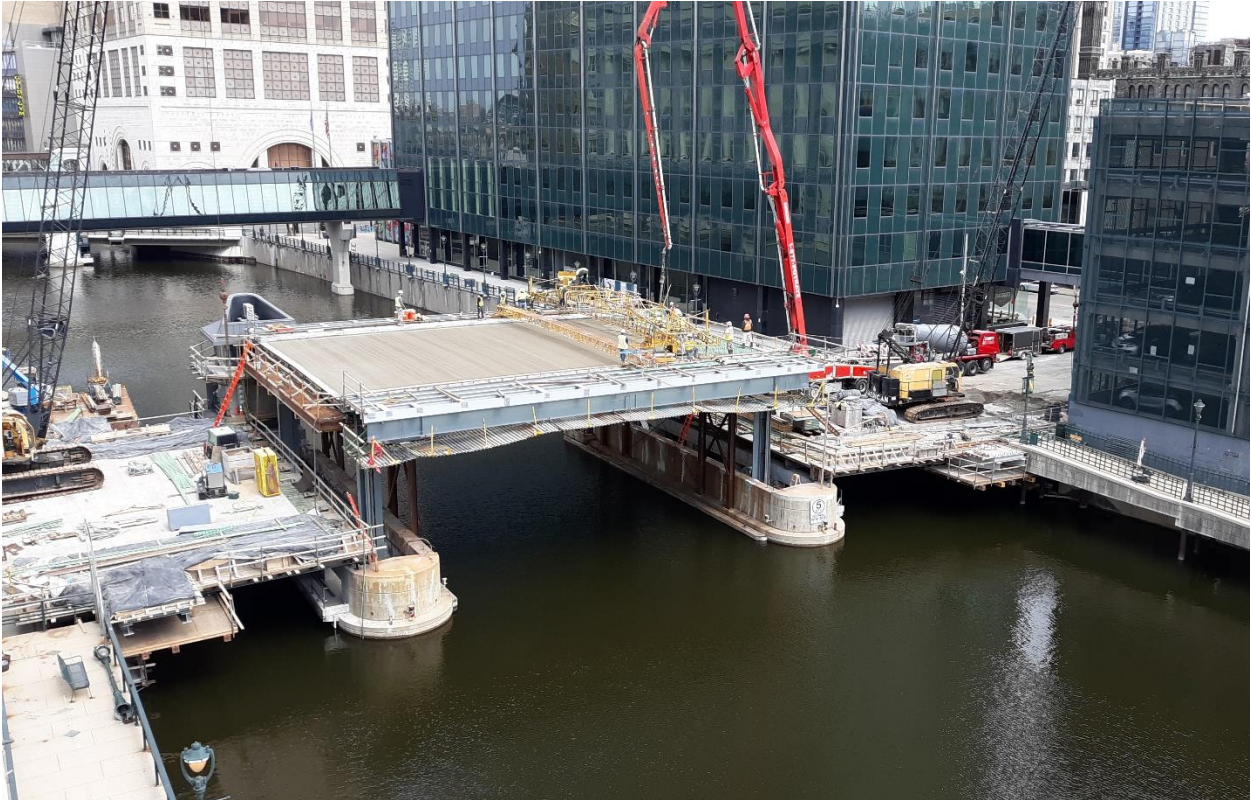
Photo 1: The Rehabilitated Bridge During the Deck Pour
