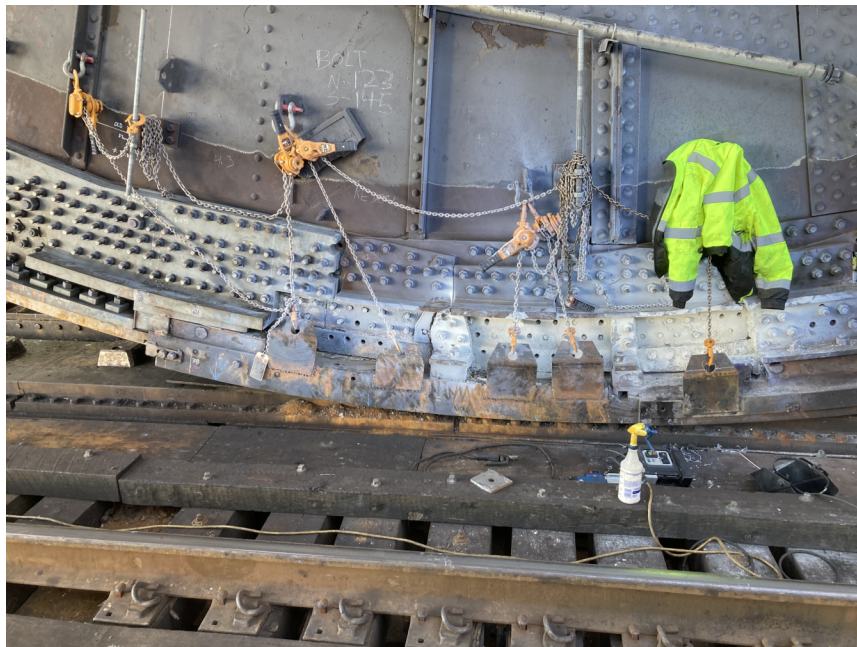
CAPTION: Pre-demo with come-alongs attached to existing tread
