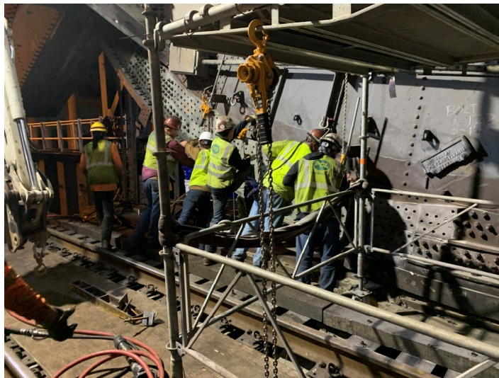
CAPTION: Drilling misaligned holes in flange angle
