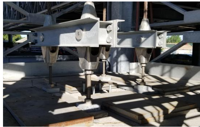
FIGURE 25: Counterweight rope connections at Macalloy bars
