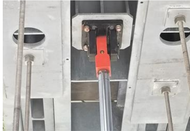
FIGURE 36: Hydraulic ram attachment to counterweight
