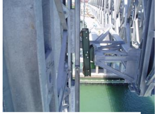
FIGURE 22: Span Guide Rollers
