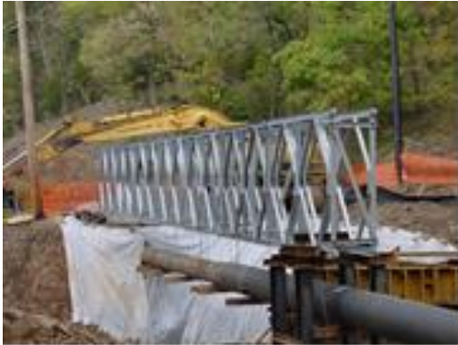
FIGURE 16: Truss bundle Support
