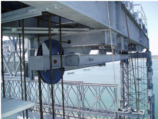
FIGURE 33: Uphaul overload device
