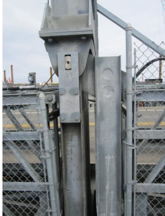
FIGURE 51: Pivot post assembly
