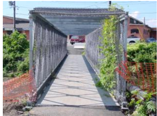
FIGURE 10: Box Pedestrian Bridge
