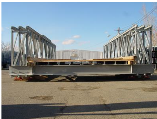
FIGURE 9: Heavy Haul timber deck
