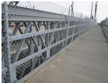
FIGURE 7: Footwalk with Fence
