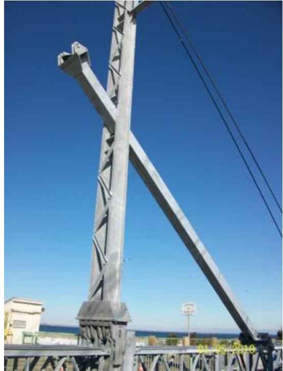
FIGURE 49: Backstay and mast assembly
