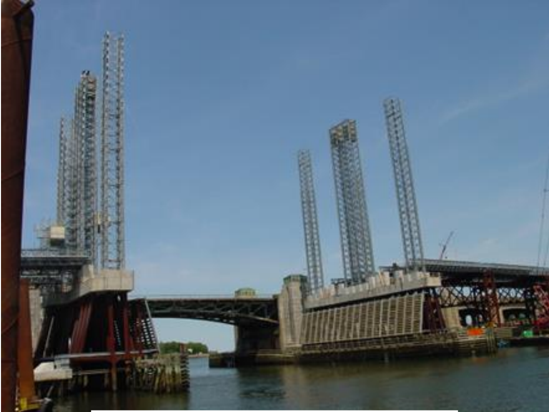
FIGURE 41: Partially installed counterweights
