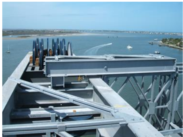
FIGURE 30: Gantry support frame at crosshead
