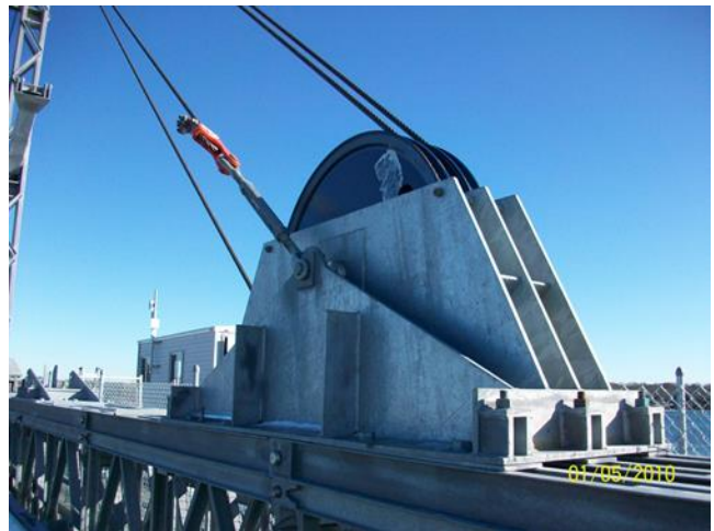
FIGURE 50: Operating rope sheave set
