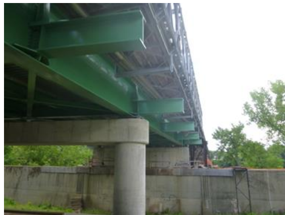
FIGURE 15: Special hangars from Pedestrian Bridge
