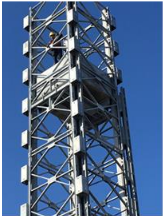
FIGURE 40: Counterweight segment installed in tower
