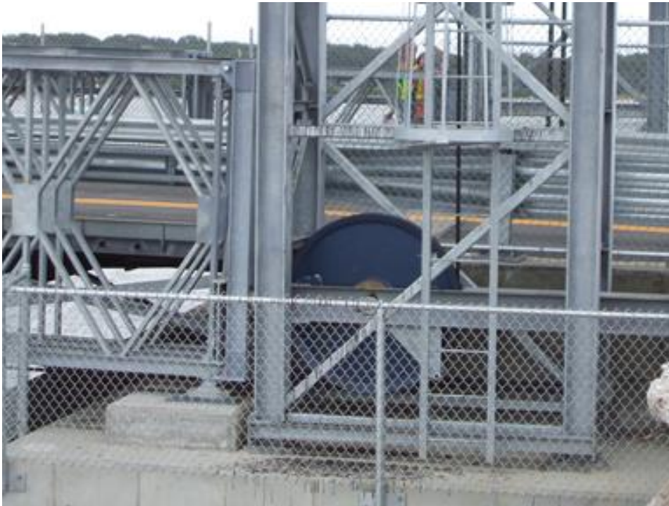
FIGURE 55: Operating rope overload protection system
