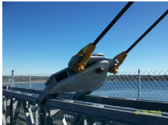
FIGURE 53: Pennant rope attachment
