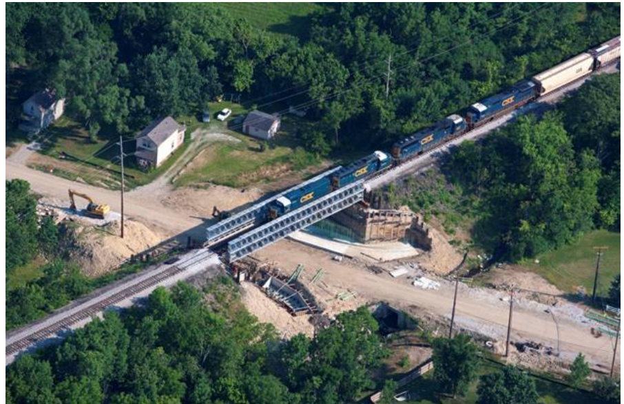
FIGURE 12: Rail bridge installation
