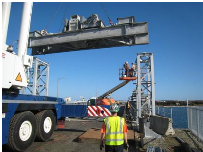
FIGURE 57: Gantry and support towers
