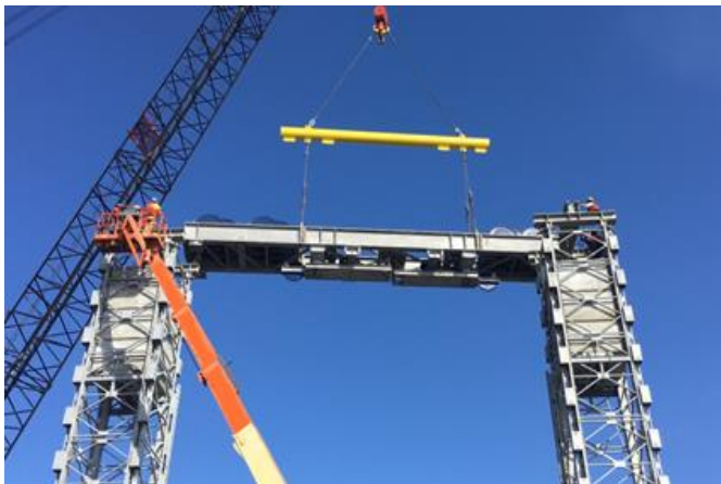
FIGURE 42: Crosshead lift-in on towers
