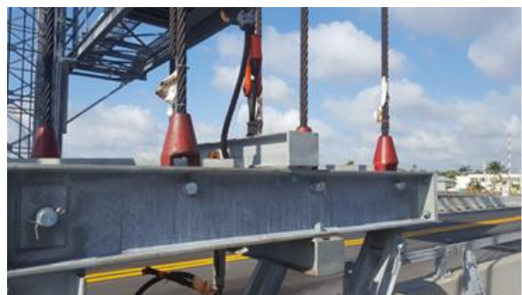
FIGURE 32: Counterweight & downhaul/uphaul rope attachments at span lifting frame
