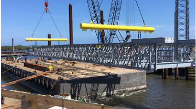
FIGURE 39: Pre-assembled gantry on barge
