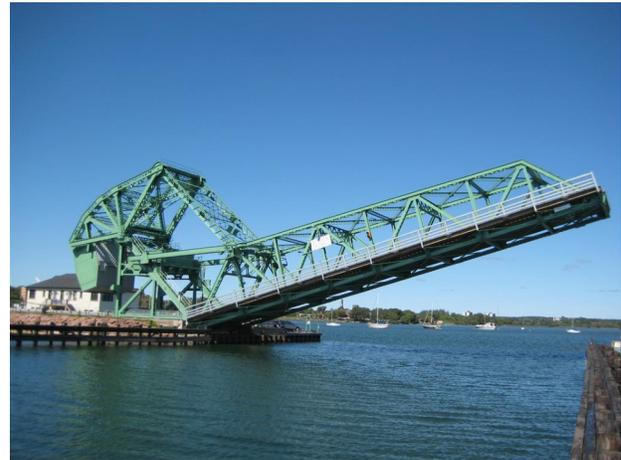
FIGURE 12: LaSalle Causeway Bascule Bridge
