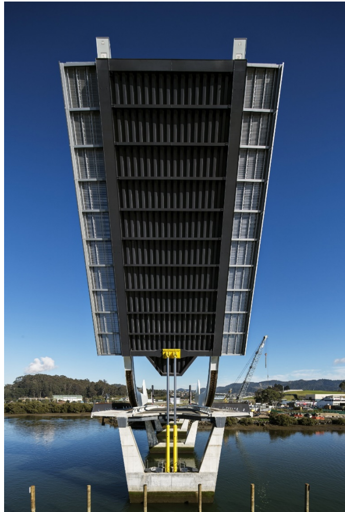
Figure 13 - Te Mata a Pohe in raised position. Note the yellow hydraulic cylinders.
