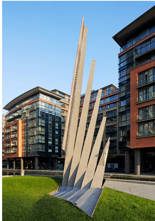
Figure 8 - Fingers in raised position. Note that the counterweights are all flush with the ground. ©Edmund Sumner
