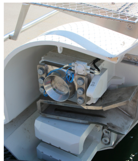
Figure 15 - Lille Langebro compression and tension sockets.
