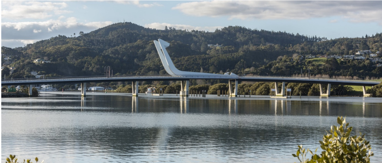
Figure 11 - Te Mata a Pohe bridge in the lowered position. ©Patrick Reynolds
