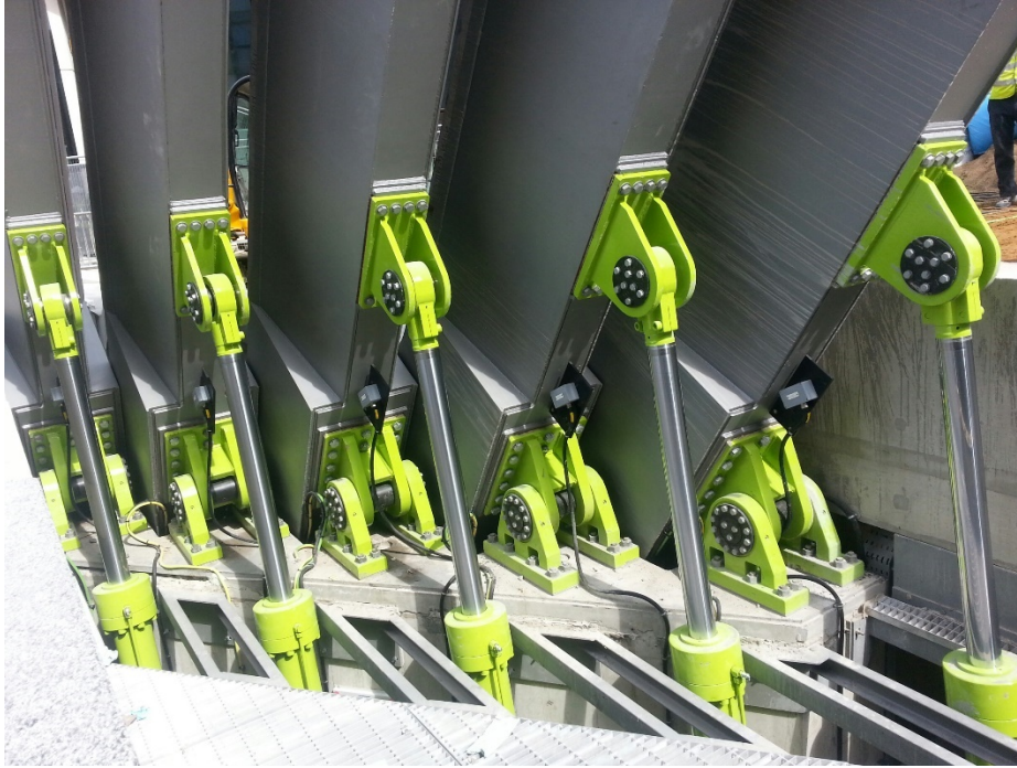
Figure 9 - Merchant Square Fan Bridge mechanisms
