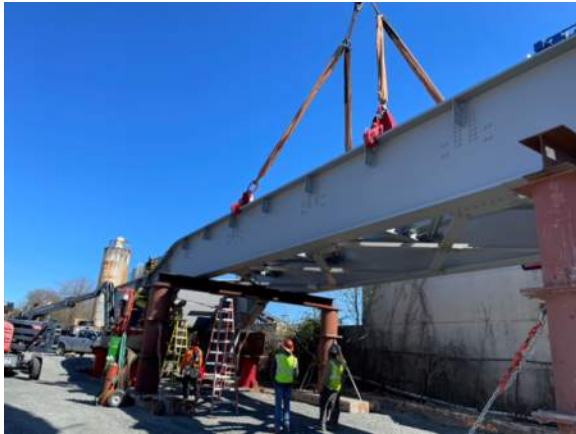
Figure 14: Leaf Assembly on the right of way. Setting the toe section (Left) and making the toe splice (Right)
