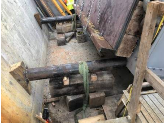
Figure 19: Restraints installed to secure the leaf in the open position.
