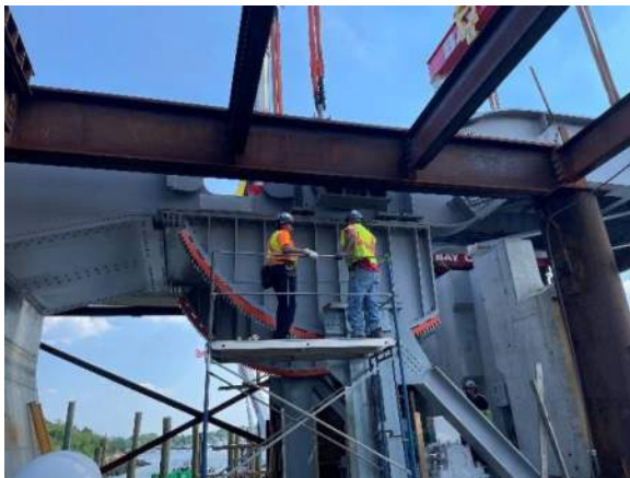
Figure 17: The leaf being lowered onto the tower (Left). The arrow indicates the alignment pin used to locate the leaf (Right).
