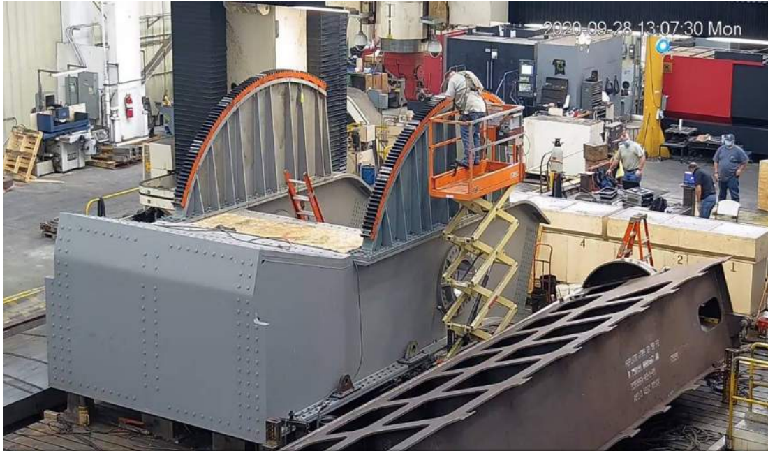
Figure 8: Screen capture during virtual shop inspection of the south bascule leaf
