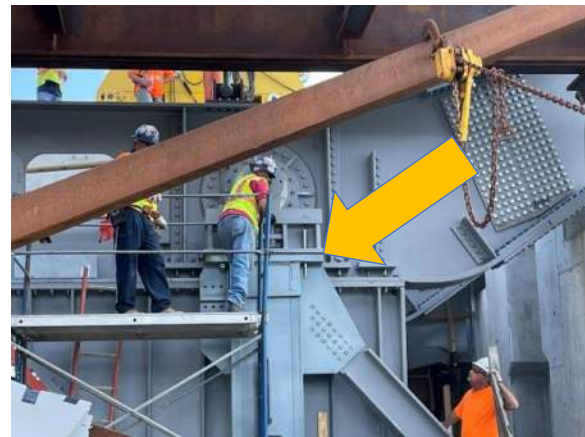
Figure 17: The leaf being lowered onto the tower (Left). The arrow indicates the alignment pin used to locate the leaf (Right).
