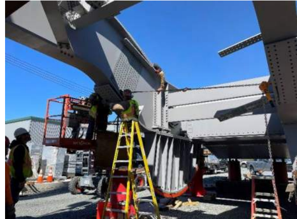
Figure 14: Leaf Assembly on the right of way. Setting the toe section (Left) and making the toe splice (Right)
