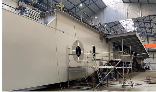
Figure 8: Bascule Girder as Fabricated
