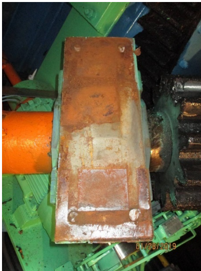
Figure 4: Bearing B1-FO. View of the failed mounting bolts remaining in the bearing base.
