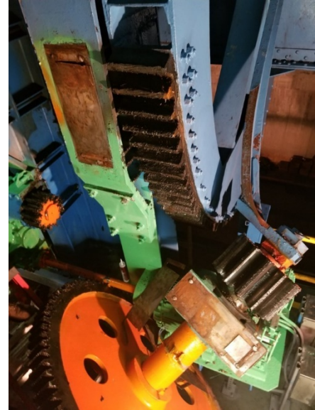
Figure 3: Unsupported rack pinion shaft resting on the motor, attached to the deformed Hopkins frame arm.
