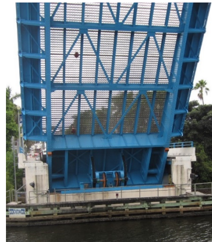
Figure 1. Representative leaf in the open position with Hopkins frame span drive machinery.
