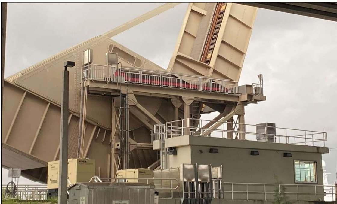
Photo 1: The CSX New River Bascule Bridge in the Open Position
