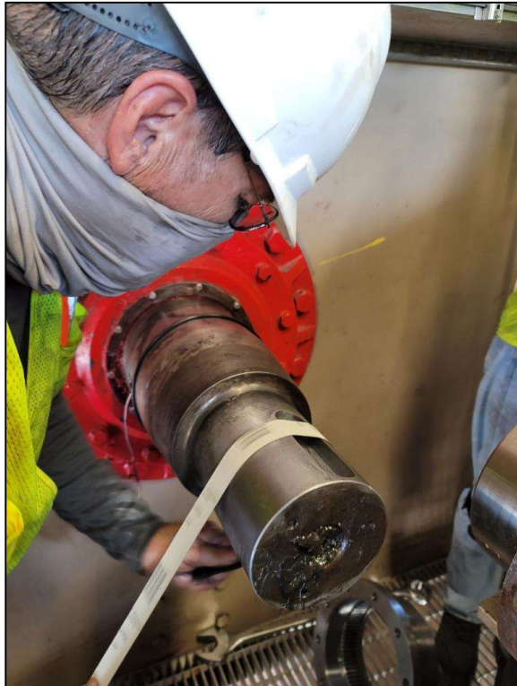
Photo 14: Millwright Polishing Shaft Surfaces
