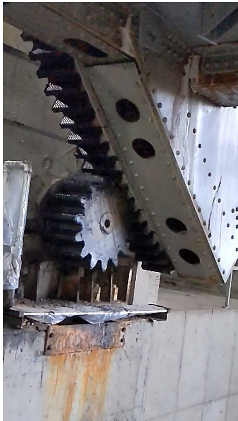
Figure 12 Morrison bascule is driven by a pinion/rack assembly on the north and south truss, 58 ft apart each other, of the bascule with the bascule structure acting as mechanical link between the two motor gear sets.
