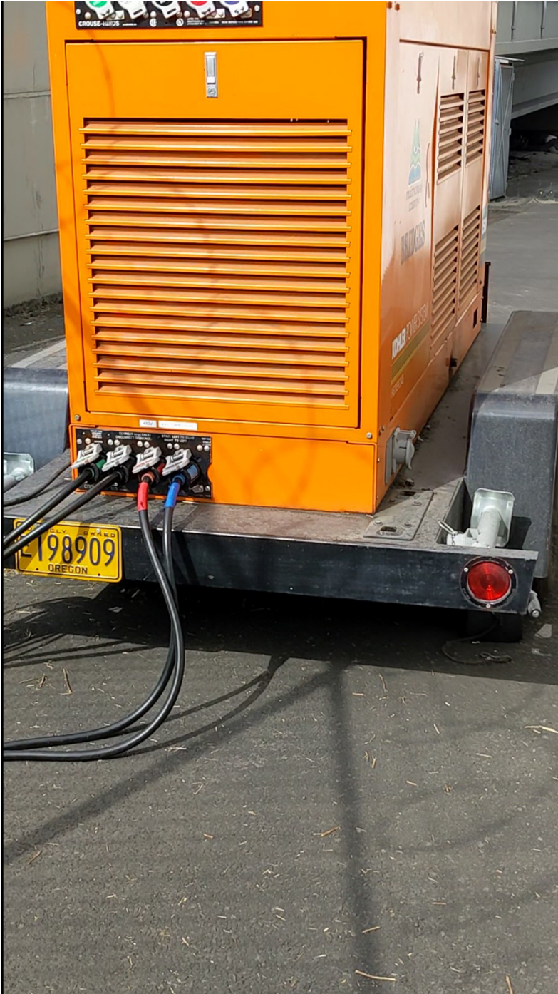
Figure 9 A very loud, 480V, diesel generator, used to power the motor drives in the shop to test motor drive/motor response. Generally, testing and troubleshooting motor drive setup and motor response required about 16 hours of generator operation.
