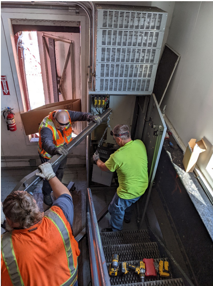
Figure 14 Fred, Mike, and Curt removing the old Broadway bridge motor drive. The external dynamic brake resister bank is on top of the motor drive electrical enclosure.
