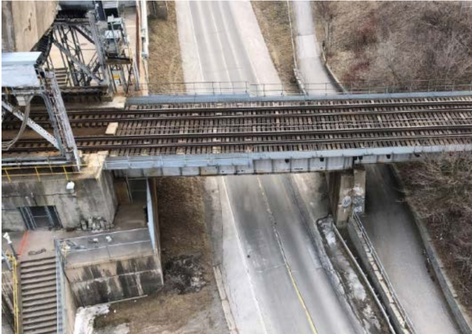
Aerial View of Bridge 6 - West fixed approach spans - (looking South)
