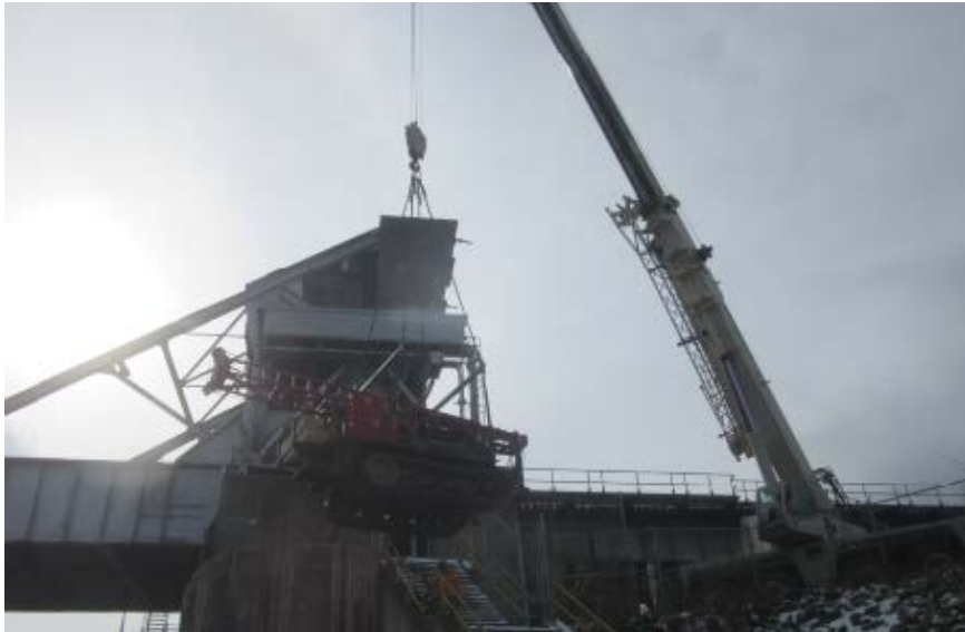
Hoisting of drill rig using 80T crane North of Bridge 6 West
