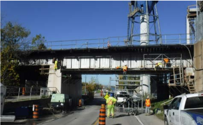
Installation of scaffolding on the South 55' span for painting work access
