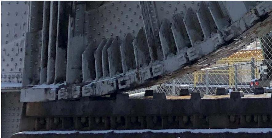
Segmental Girder flange reinforcing gussets (Left picture) and Tread Plate pocket mechanical splints (Right picture)
