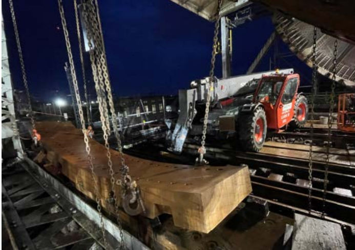
Installation of new front tread
