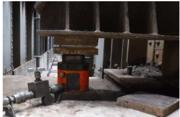
South 35' span jacking for the replacement of the bearing plates
