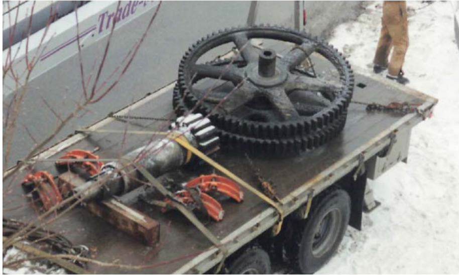
Bridge 6 mechanical drive refurbishment project in early 2000's
