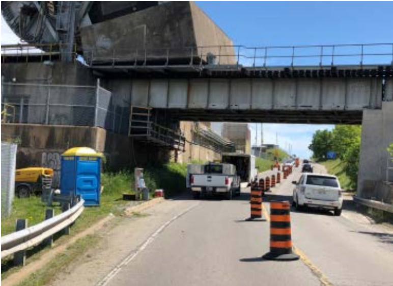
Fixed Approach Spans Center Pier Rehabilitation completed – southbound lane re-opened
