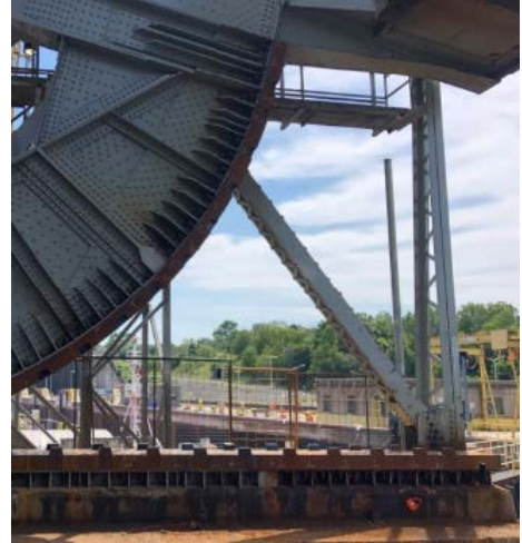
Track plate segments (South) East span shown – raised - West side similar
