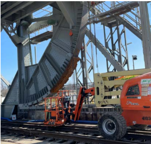
Installation of new middle and back tread
