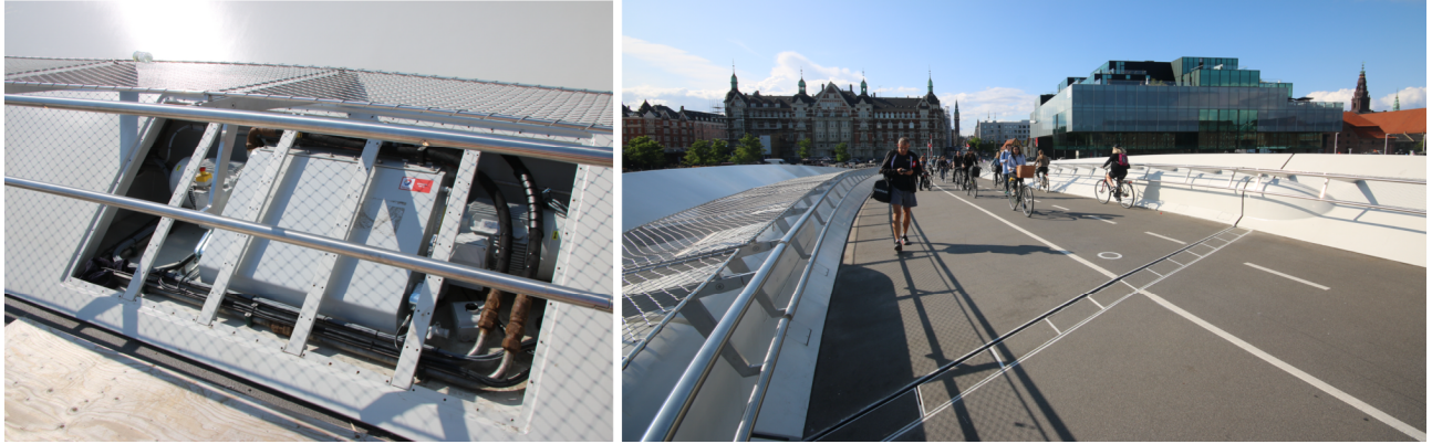
Fig. 8. Hydraulic power pack within main beam (L). 'blisters' in beams at joint (R). Source: Eadon Consulting
