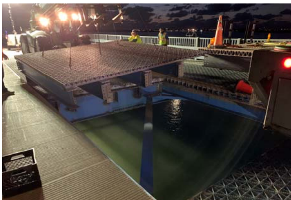
Figure 11. Existing Deck and Stringer Removal
