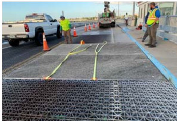
Figure 12. Prototype Panel Installed
