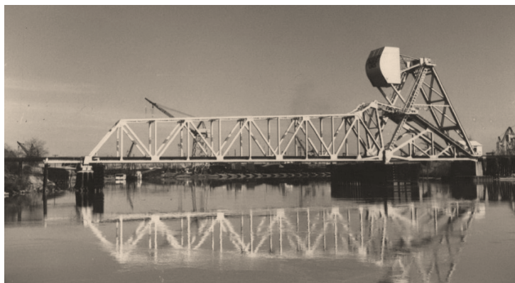
Figure 1 - 230-ft Span at Beaumont Texas
