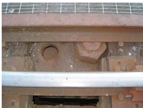
Figure 8 – The bolt to the right of the open hole was also identified to be failed.
