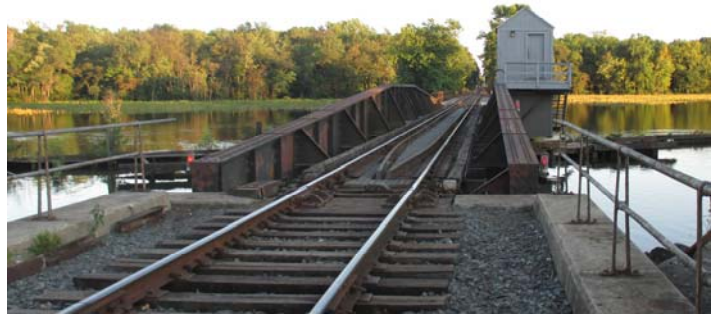
Figure 2: View of swing span from south approach. The span is aligned and supported for rail traffic.
