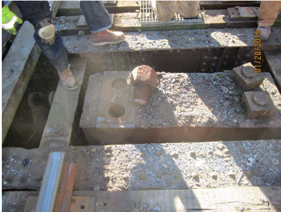
Figure 15 As-Found Condition of Center Support Assembly. (after removal of rail and ties)
