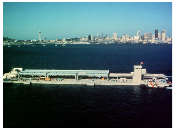
Figure 4. East Half Draw Leaving the Graving Dock.
