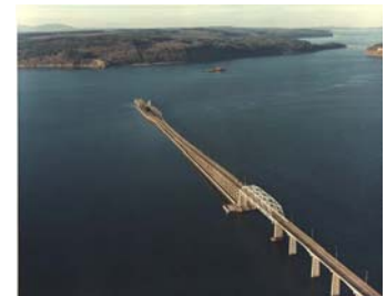
Figure 2. Hood Canal Bridge after West Half Sunk
