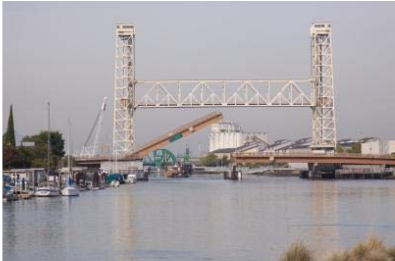
Alameda County, CA - ABL-Fruitvale Tower Drive Vertical Lift Bridge over Oakland Inner Harbor.
