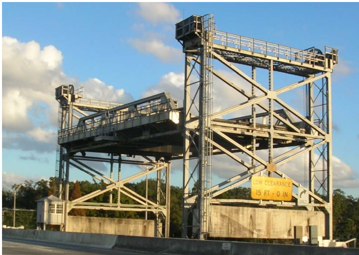
FIGURE 21 - Span Stuck in Open Position
