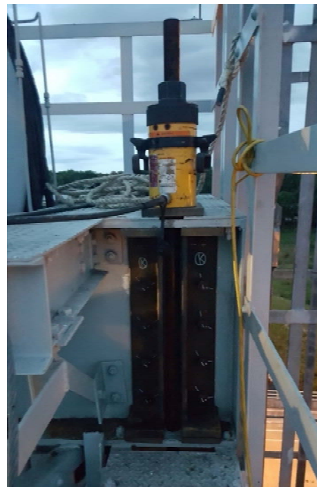
FIGURE 23 - Screw Jack with Tie-Rod and Stiffeners
