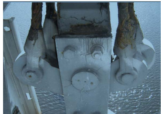
FIGURE 25 - Original Counterweight Connection Assembly
