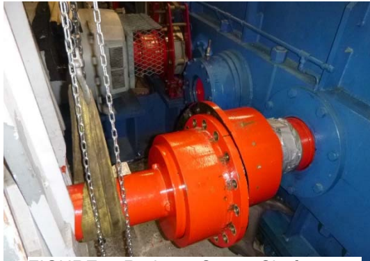
FIGURE 5: Reducer Output Shaft Coupling Disconnected
