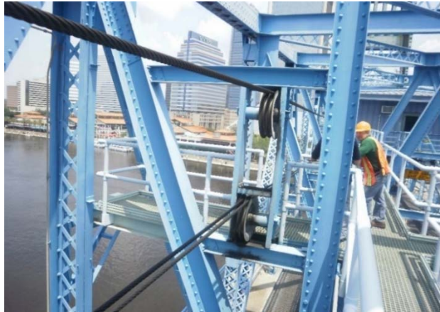
FIGURE 8: Operating Ropes Through Idler Sheaves
