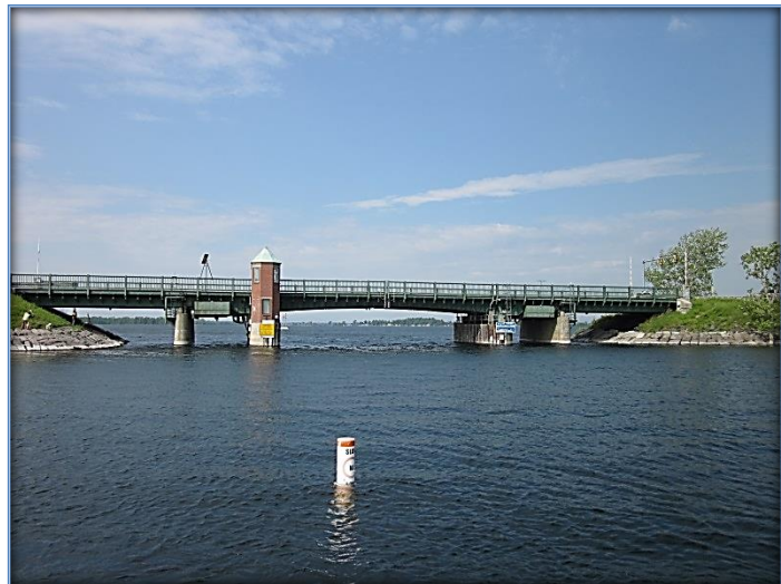
Elevation View of the Existing North Hero Bridge
