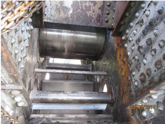
Photo 23: View inside the counterweight truss as the existing sleeve was lifted out of position. Temporary bracing installed as the sleeve moves along the removal path.
