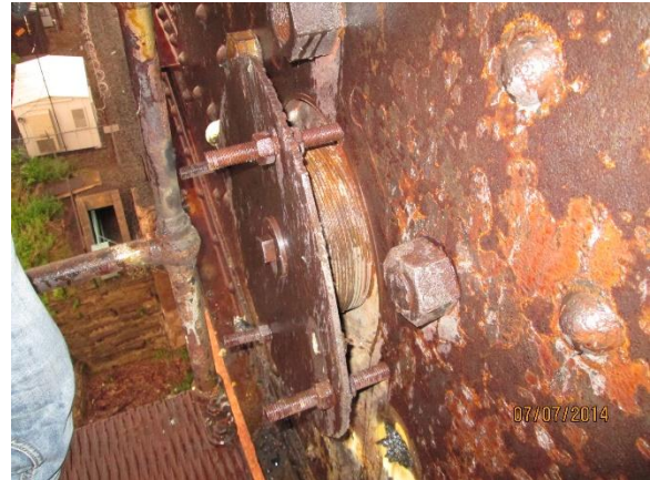
Photo 4: North Counterweight Trunnion Bearing, Outboard. The pin nut is missing which has allowed the pin to move axially to the south.
