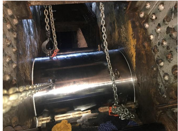
Photo 32: The new sleeve hung in place inside the counterweight truss, aligned to the bushing.
