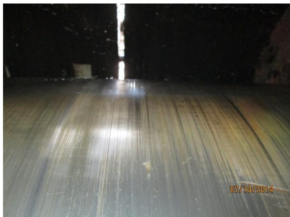
Photo 9: North Counterweight Trunnion Bearing, Span Open. There is light bronze embedment and corrosion where the trunnion sleeve makes contact with the lower half of the bearing.
