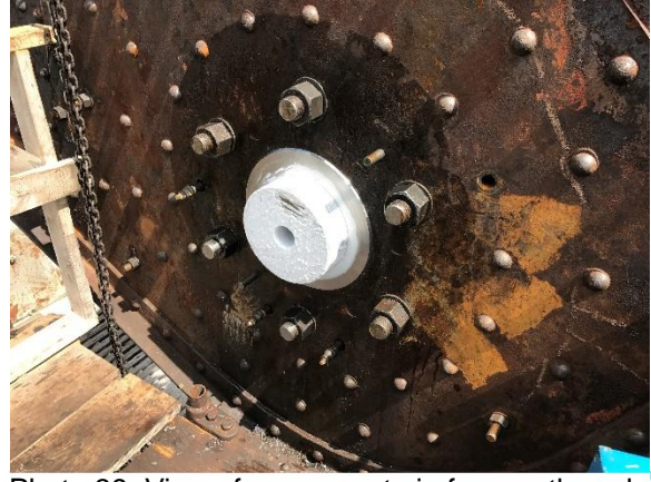
Photo 39: View of permanent pin from outboard side after it was fully inserted, prior to installation of the pin nut.
