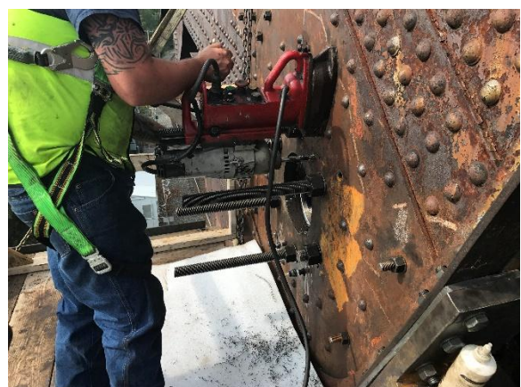
Photo 34: Drilling holes for alignment dowels.
