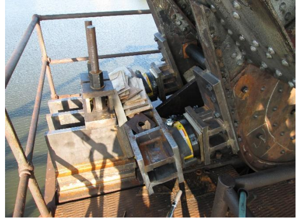
Photo 21: Horizontal jacking system installed.
