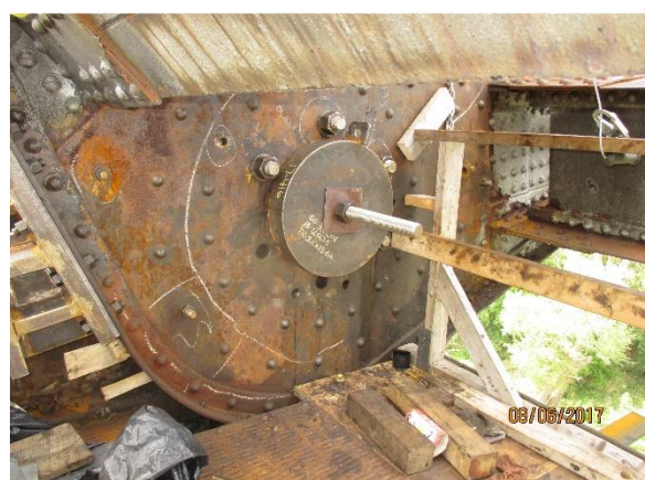
Photo 28: Temporary pin secured, work window 1 complete.
