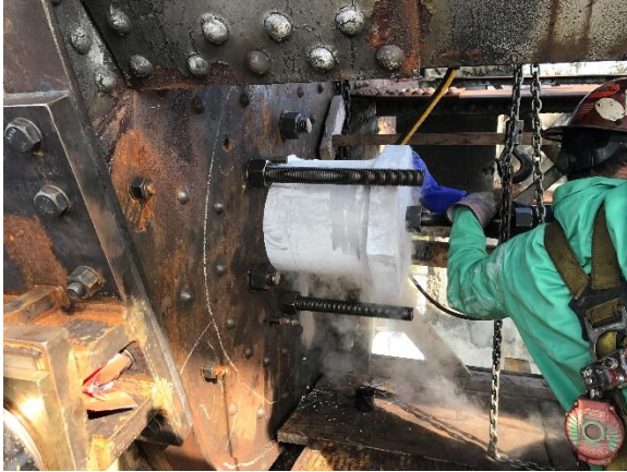
Photo 38: Permanent pin partially installed from inboard side of truss.
