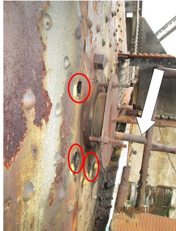
Photo 7: North Counterweight Trunnion Bearing. Five of six turned studs which secure the trunnion sleeve to the counterweight truss plates are sheared and are either missing (3 red circles, one not visible) or are protruding from the assembly (arrow).
