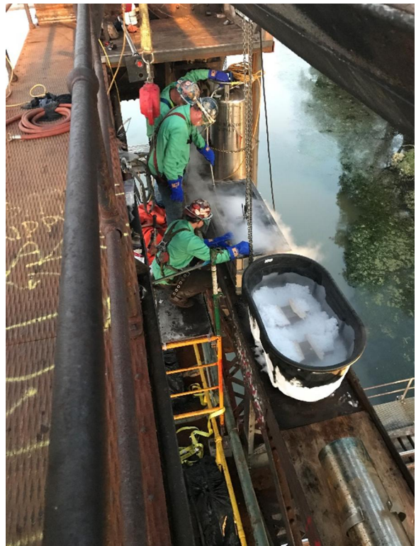
Photo 37: The permanent pin has been removed from the dry ice and transitioned to the liquid nitrogen for further cooling.
