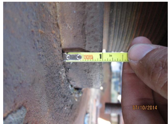
Photo 5: North Counterweight Trunnion Bearing, Inboard. Close up of the bearing pin revealing axial movement 1" to the south.
