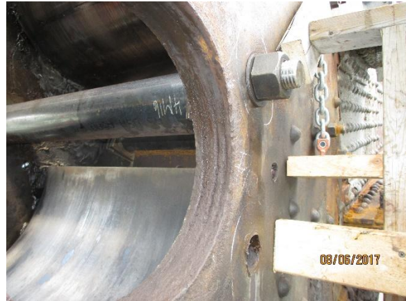
Photo 24: Close-up view of the wear/damage/corrosion on the inboard truss gusset plate where it bears on the pin.
