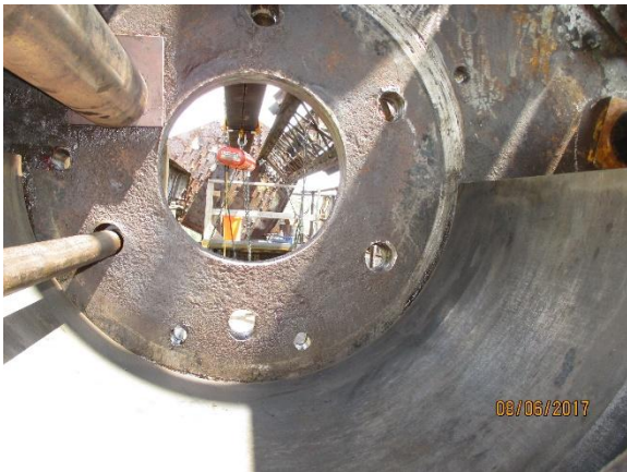
Photo 25: View inside the counterweight truss with the bushing removed and the existing bearing housing cleaned for inspection and measurement.
