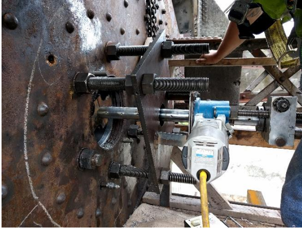
Photo 35: Line boring equipment installed and boring underway.
