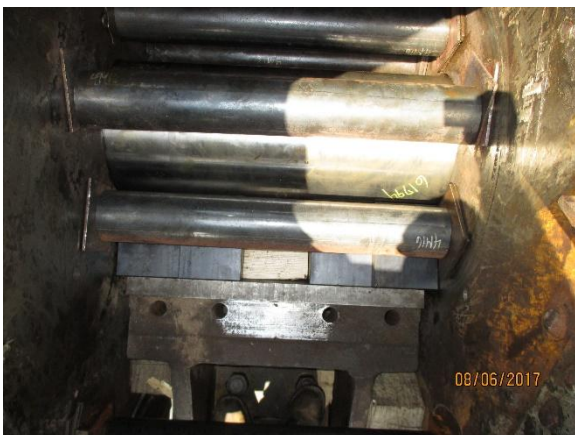
Photo 27: View inside the counterweight truss with the engineered plastic "quarter-sleeve" blocking system installed and the temporary pin in place.
