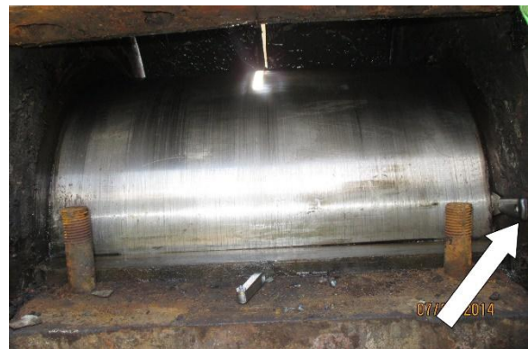
Photo 10: North Counterweight Trunnion Bearing, Span Closed. When viewed from the counterweight side of the bearing, there are gaps between the sleeve and the truss plates. A scraper has been inserted in the gap between the outboard end of the sleeve and the truss (arrow).
