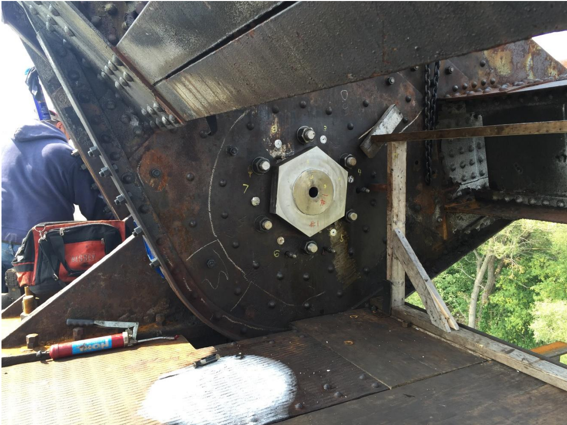
Photo 42: View of completed repair from inboard side of the counterweight truss.
