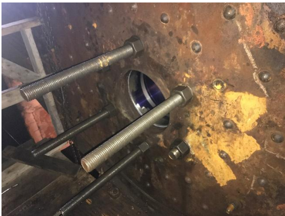
Photo 33: Temporary studs installed and tensioned to secure the new sleeve.
