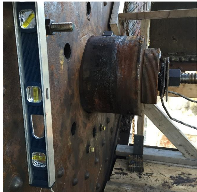
Photo 22: Close-up view of the existing counterweight trunnion pin where it interfaces with the counterweight truss during removal.
