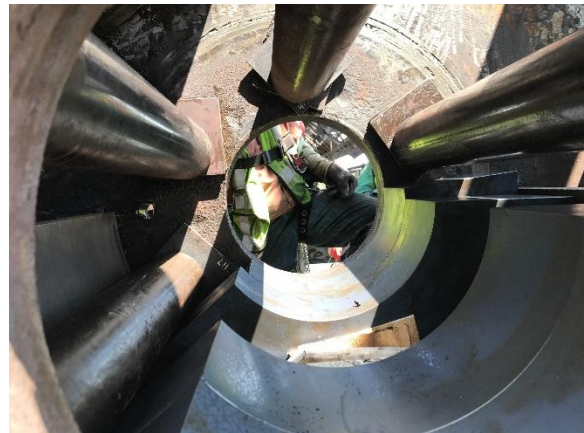
Photo 26: View inside the counterweight truss with the engineered plastic "quarter-sleeve" blocking system installed prior to installing the temporary pin.
