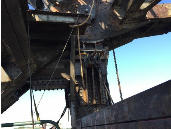
Photo 20: Vertical jacking system installed.
