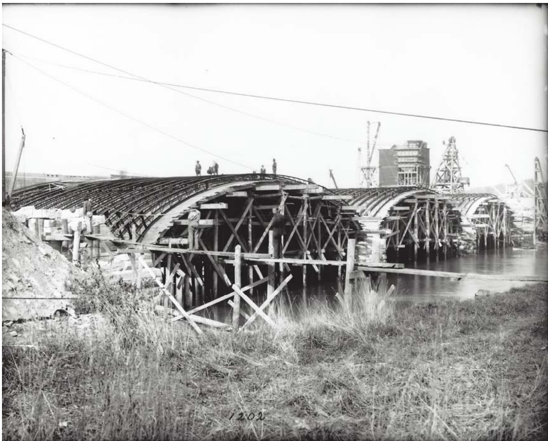
Pelham Bridge Concrete Arch Construction using the Melan System
