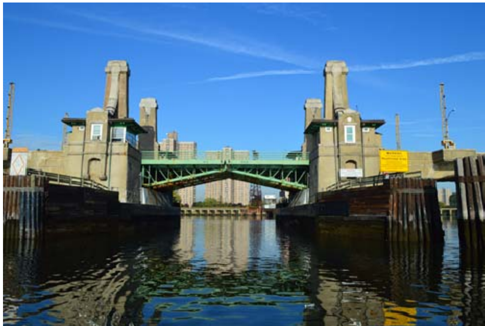
Existing Shore Road (Pelham) Bridge
