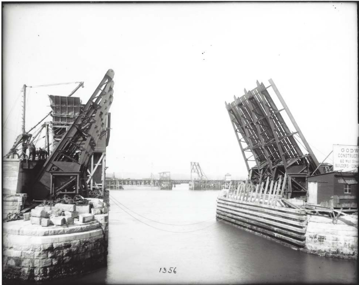
Pelham Bridge Scherzer Span Under Construction
