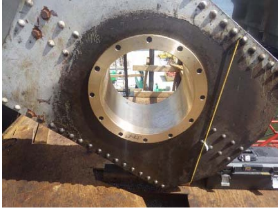
Photograph 8 - New bushing in the lakeside counterweight link bearing
