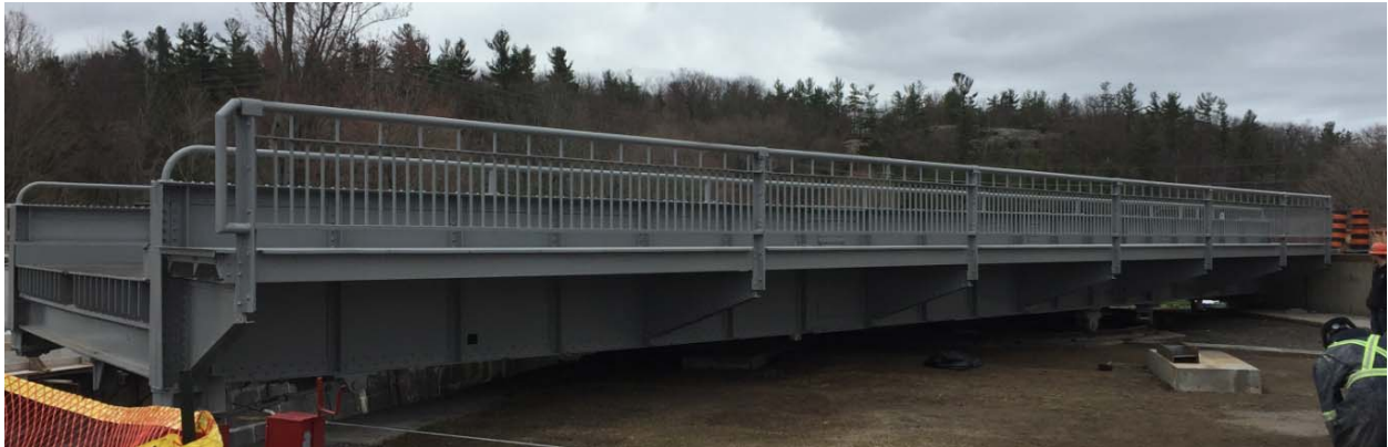
Figure 14: Kingston Mills Swing Bridge
