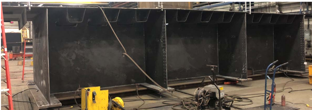
Figure 6: Central pivot - Brighton swing bridge
