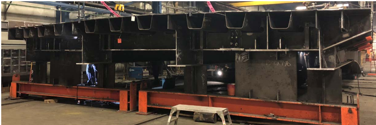
Figure 5: Completed pre-assembly of the Brighton swing bridge
