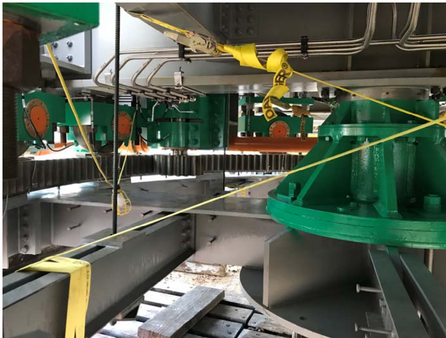
Figure 12 Grillage Frame and Machinery Aligned and Secured Prior to Float-In
