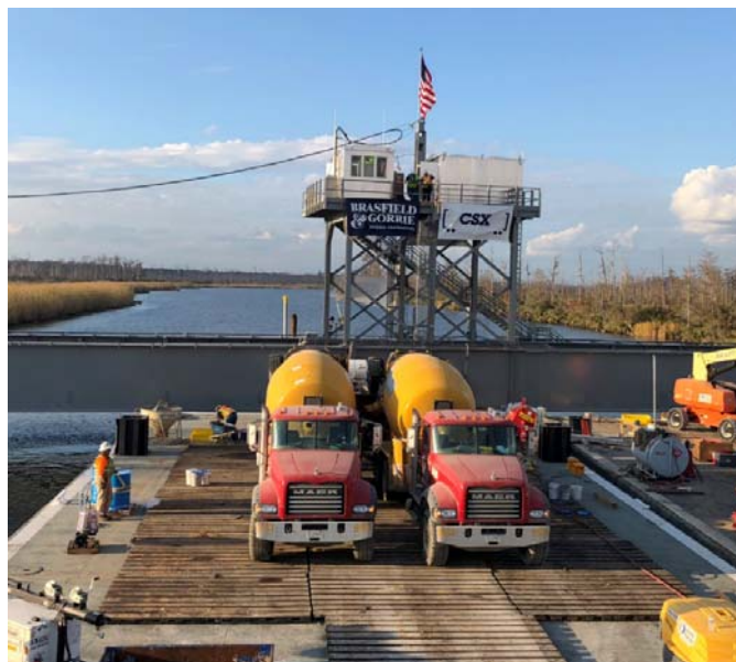
Figure 21 Barge and Concrete Truck Setup
