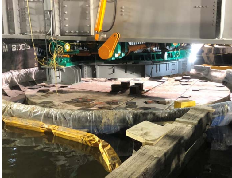
Figure 19 Grillage Alignment Over Center Pier Shims
