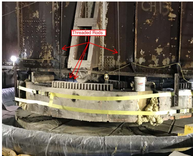
Figure 16 Existing Center Pier Cap Removal
