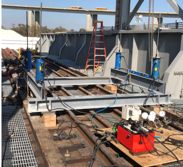
Figure 11 Grillage Jacking Frame
