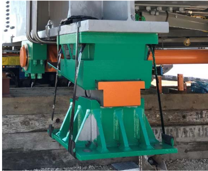
Figure 13 End Wedge Installation Prior to Float-In
