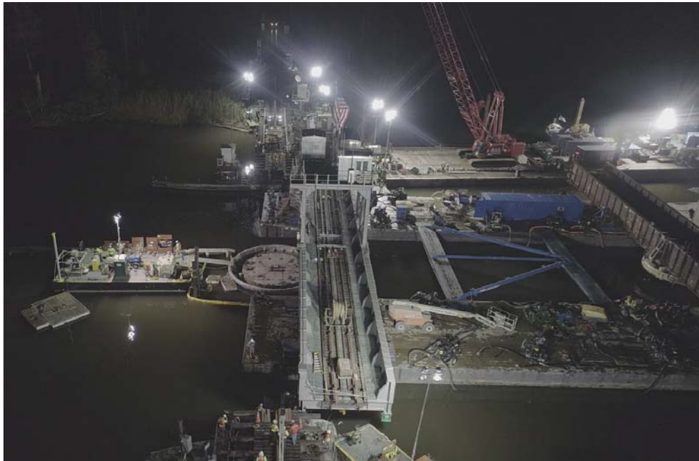
Figure 18 Bridge Float-In Over Existing Piers
