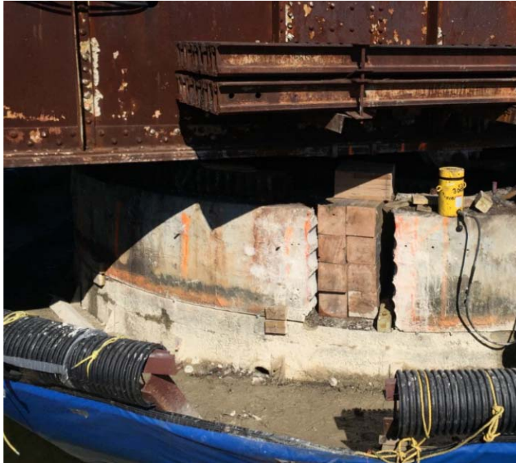
Figure 8 Timber Blocking in Pocket
