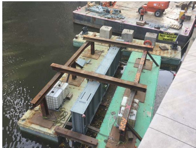
Figure 10: Flexifloat barge with Longitudinal Girder
