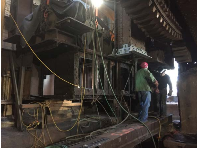
Figure 9: Trunnion Column and Machinery Girder
