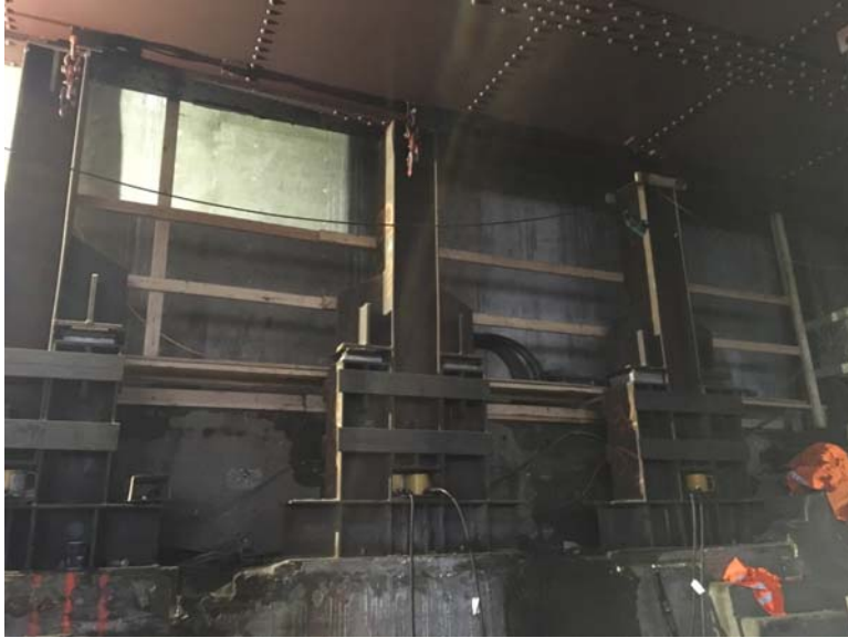
Figure 5: Shoring Towers for Counterweight Box
