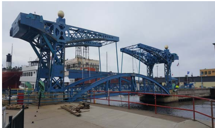
FIGURE 1: View of Minnesota Slip Pedestrian Bridge looking Northeast.
