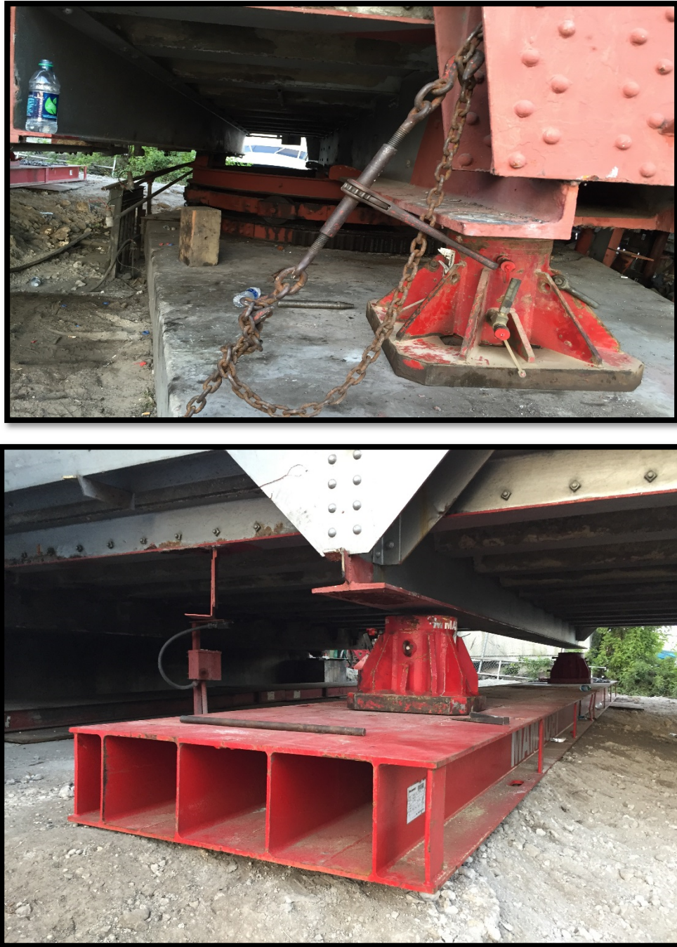
Figure-5: Climbing Jack position underneath the beam and on the Load spreader beam
