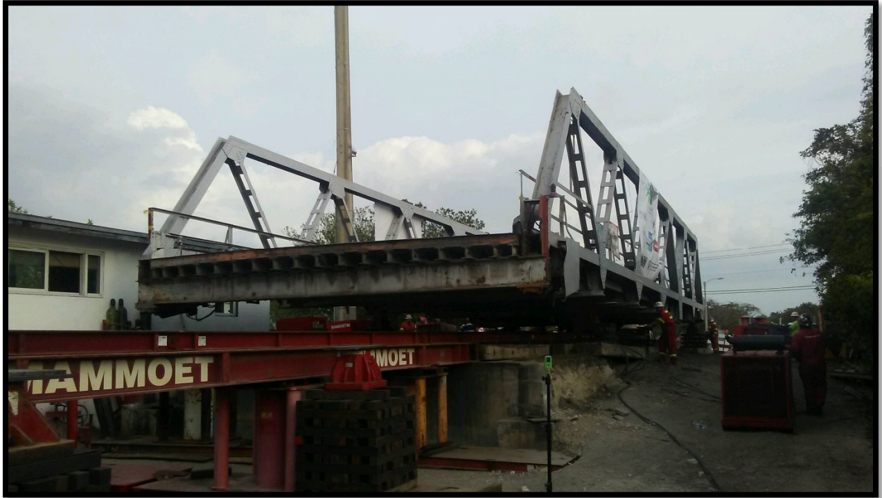
Figure-11: Project Photo of Bridge Skidding
