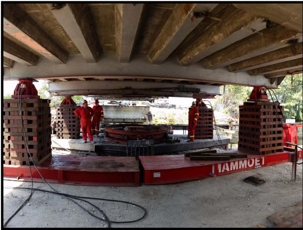
Figure-7: Project Photo of Jacked up Bridge
