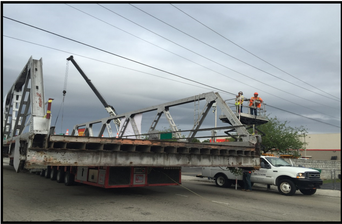
Figure-14: Utility check as bridge goes through streets
