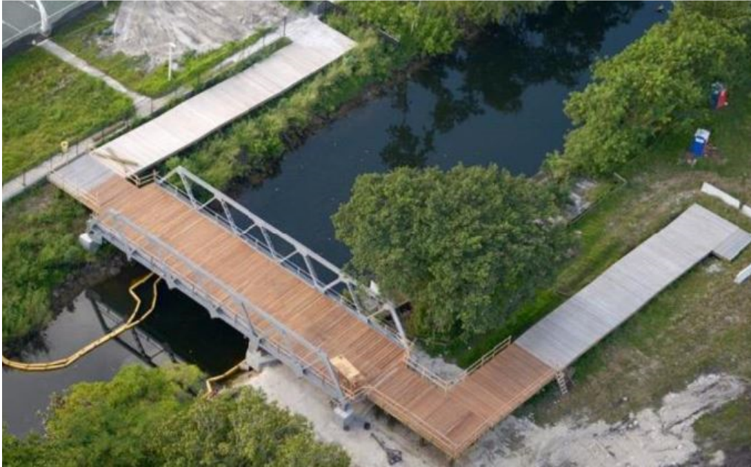
Figure-15: Bridge restored at new location (as pedestrian bridge)
