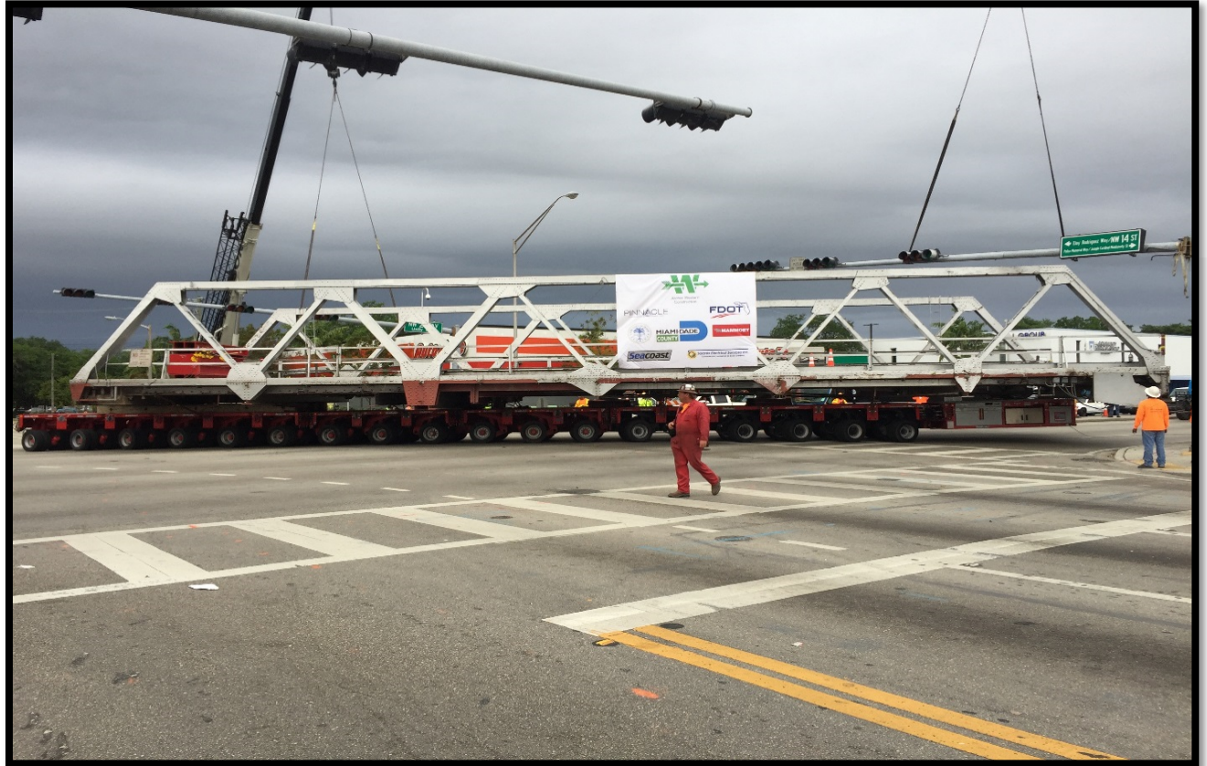
Figure-1: Bridge on SPMT at Junction of NW 27 th Ave. & NW 14 th Street
