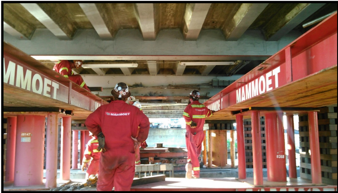
Figure-9: Project Photo of Skidding System installation
