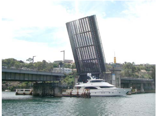
Photograph 1 – General view of the Spit Bridge
