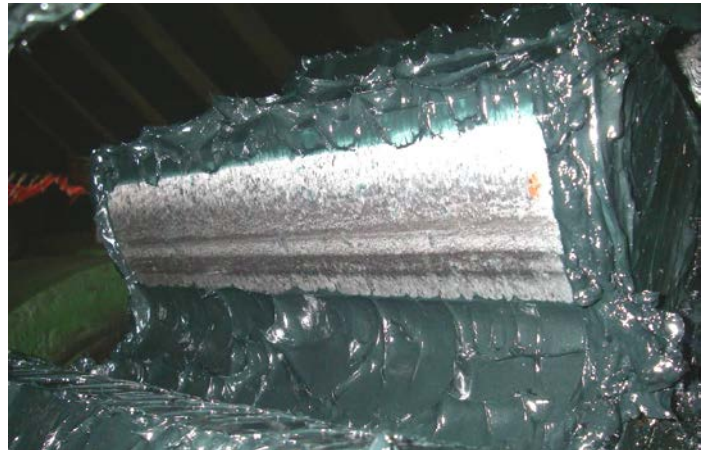
Photograph 3 – East pinion contact pattern prior to grease removal.
