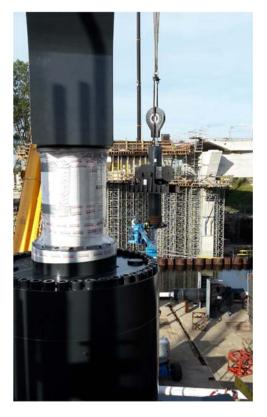
After this operation was done, the bridge was ready to be installed. Also this operation was done with a floating carrier and took 1 day per bridge (including filling the counter weight). After installation of the bridges, the coupling of the hydraulic cylinders with the bridge took place.
